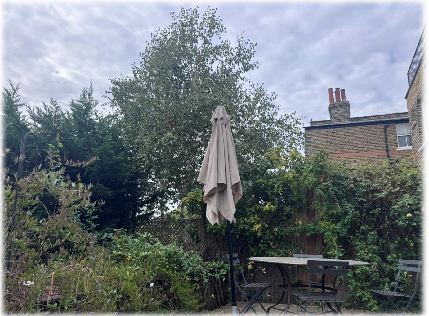
Exiting Raised Terrace with – Large Retaining Wall on left Side of Terrace Acting as a Root Barrier Deflecting any Tree Roots
