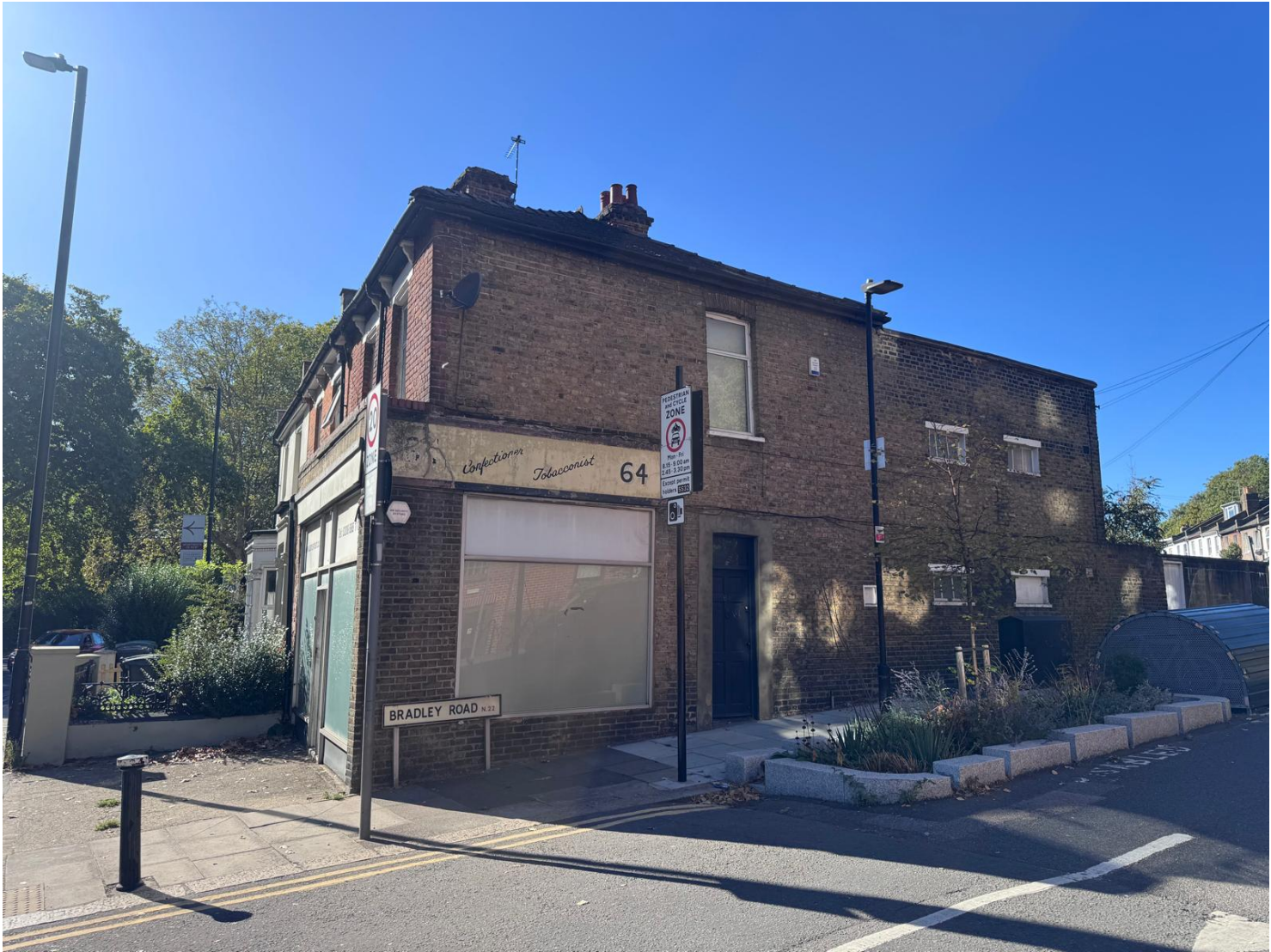
View - Bradley Road
