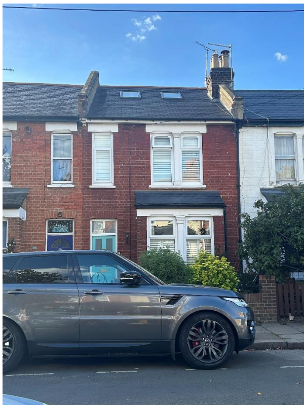
Existing front elevation view
