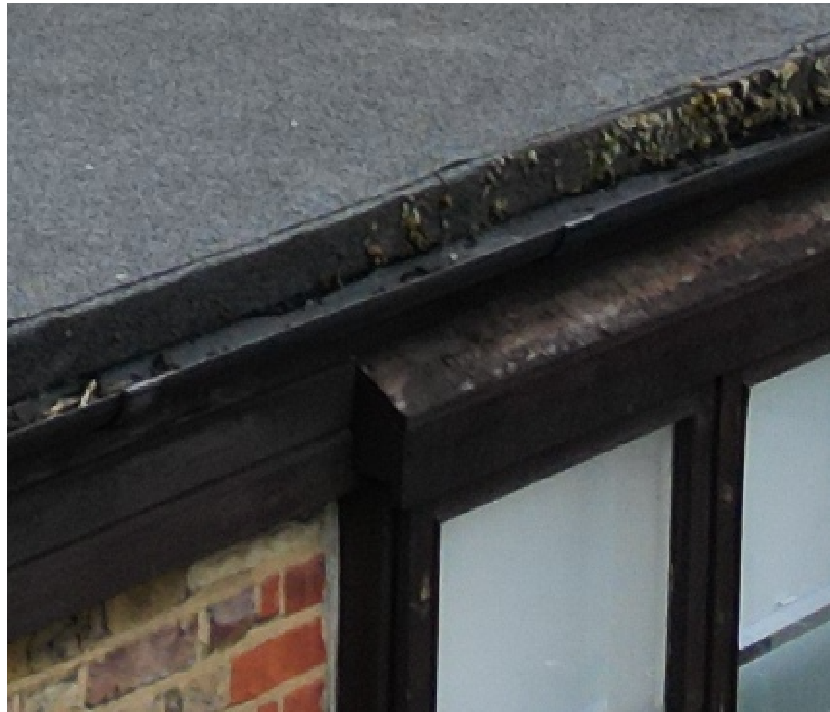
existing fascia & windows
