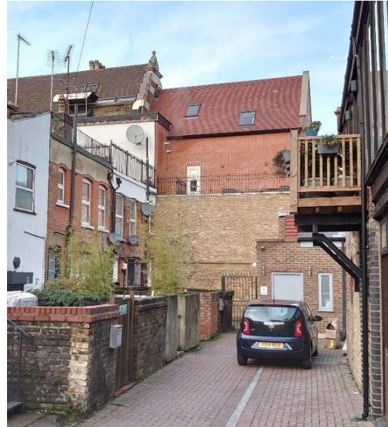
View towards 1 Rose Place and rear of properties on The Broadway
