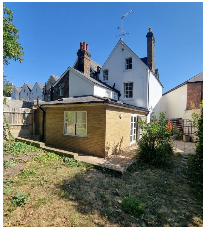
View of rear elevation
