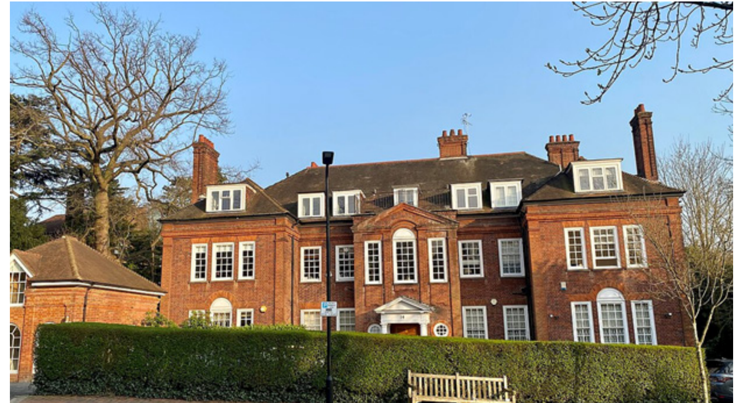
14 Templewood Avenue, Hampstead, designed by Quennell between 1910-11. The timber entrance portico is centred on the front gable which is also what we propose for the new entrance to Derwen.
