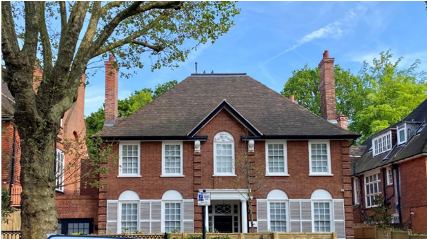
24 Heath Drive, Hampstead, designed by Quennell in 1907. The timber entrance portico and detailing to the front door is to be replicated in the design of the new front entrance to Derwen. Note the entrance portico is centred on the front gable.
