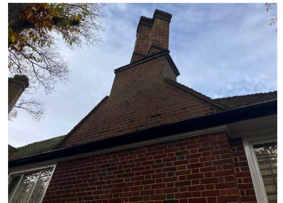
Existing chimneys will be retained in their original form
