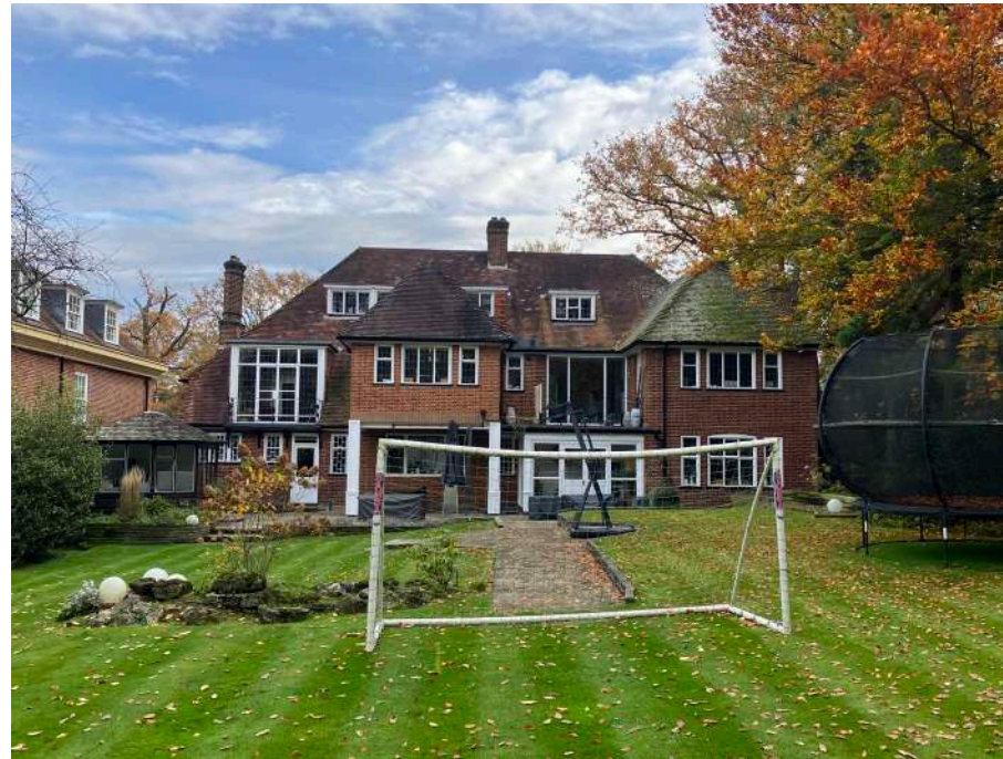
Rear Elevation of the existing property -has already been modified over the years
