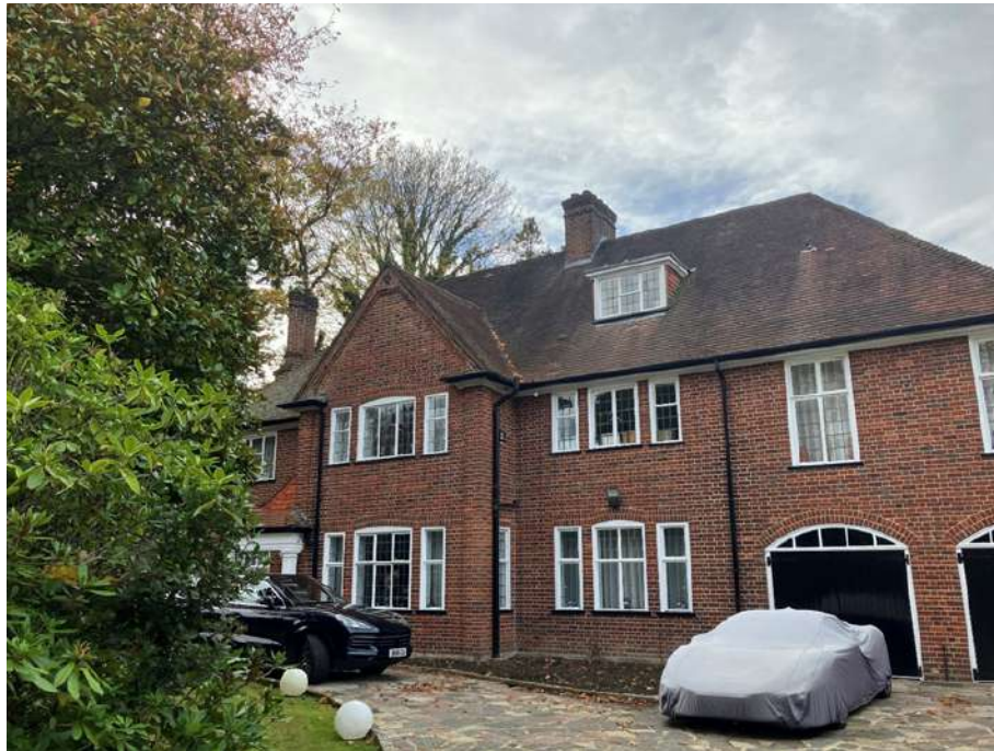
Front Elevation of the existing property - to be retained and modified
