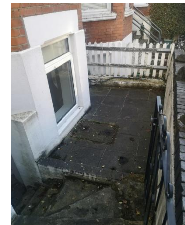
Front area of upper grd basement & ground level front wall
