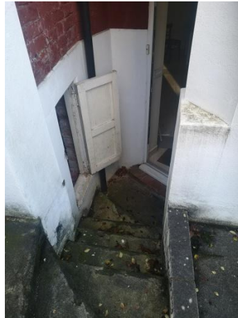
Cement steps down to Lower Grd Basement and Meter Cupboard
