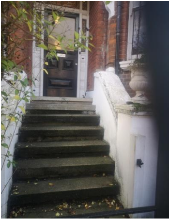
Front Cement Steps to Front Door
