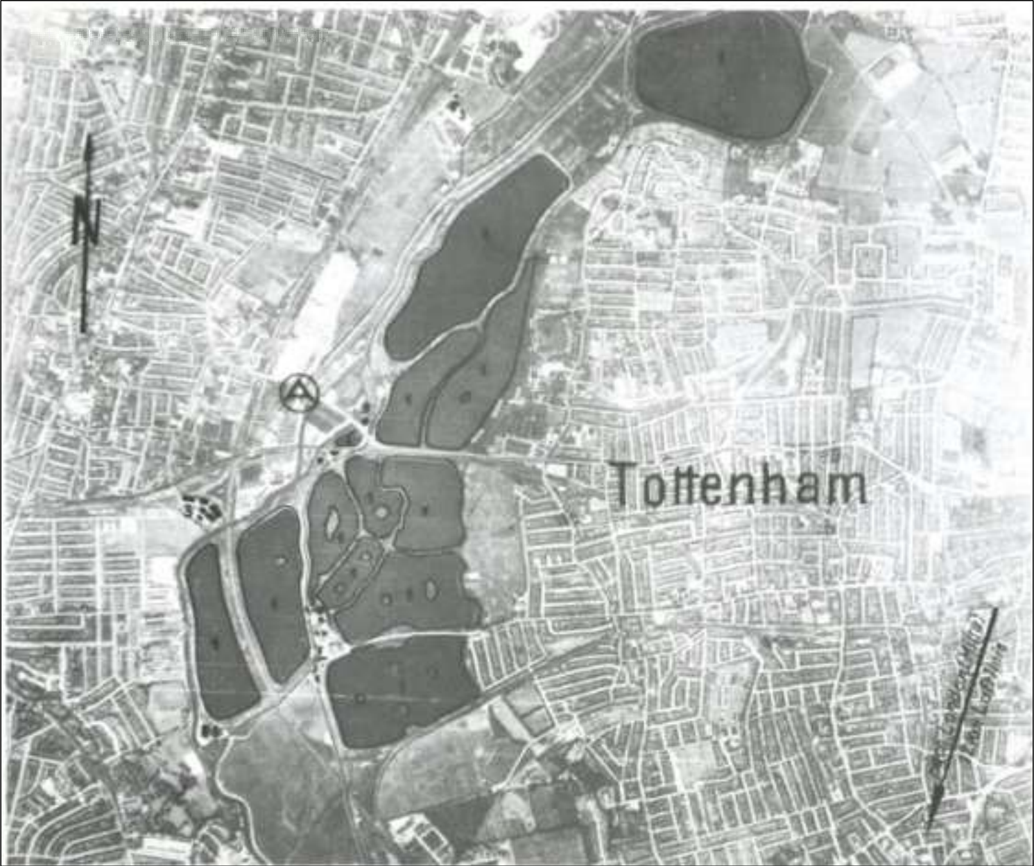
London – Tottenham A. Water Treatment Works and Reservoir
