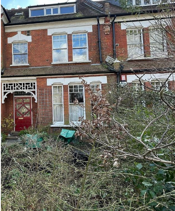
Down pipes from shared roof line
