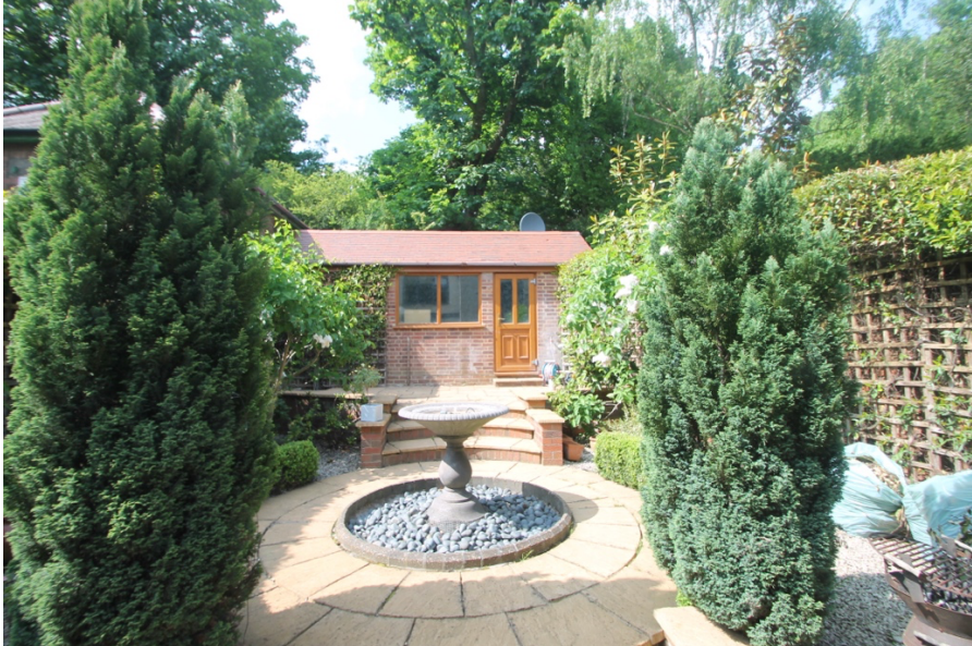
Garage. Elevation viewed from rear garden of 100 Priory Gardens
