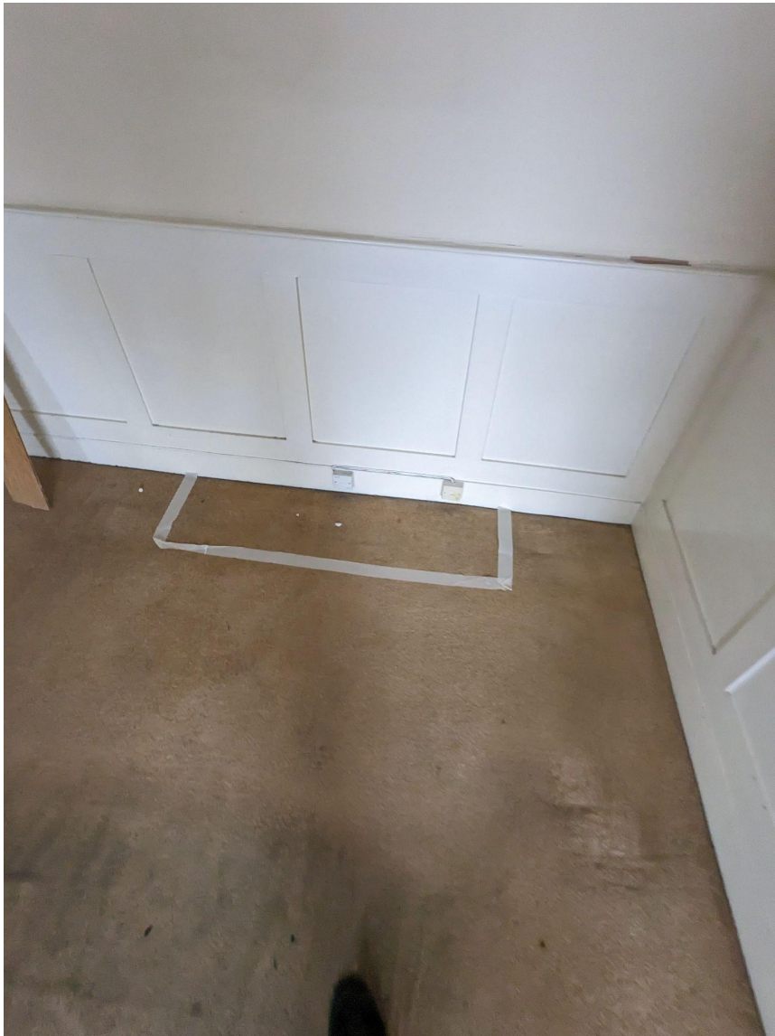
Internal view of timber panelling
