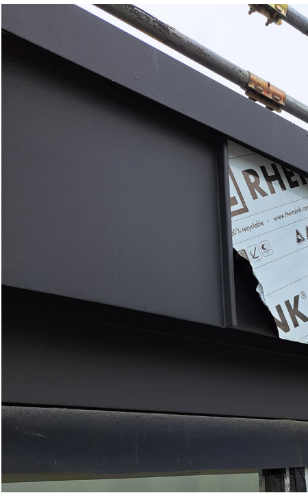
New Zinc flashing as part of RFS-501 shown above and to left on slate roof - matching existing construction and style of existing roof
