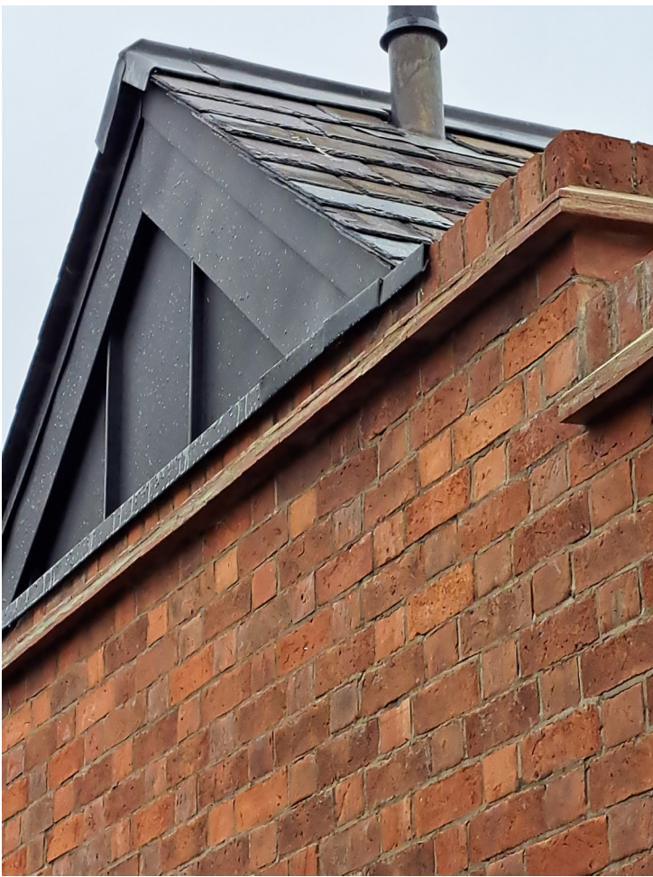
New Zinc flashing as part of RFS-501 shown above and to left on slate roof - matching existing construction and style of existing roof
