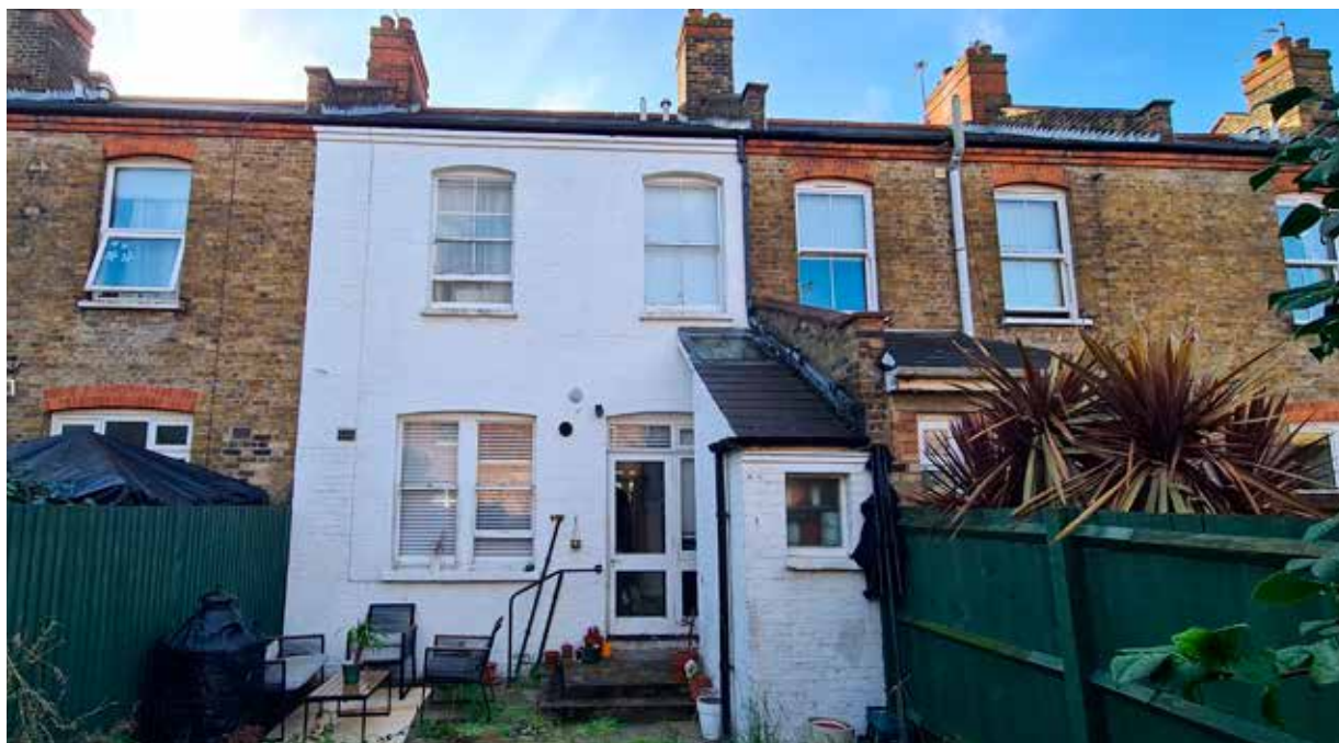
Photo 3 - Rear of the house painted white with the small lean-to extension
