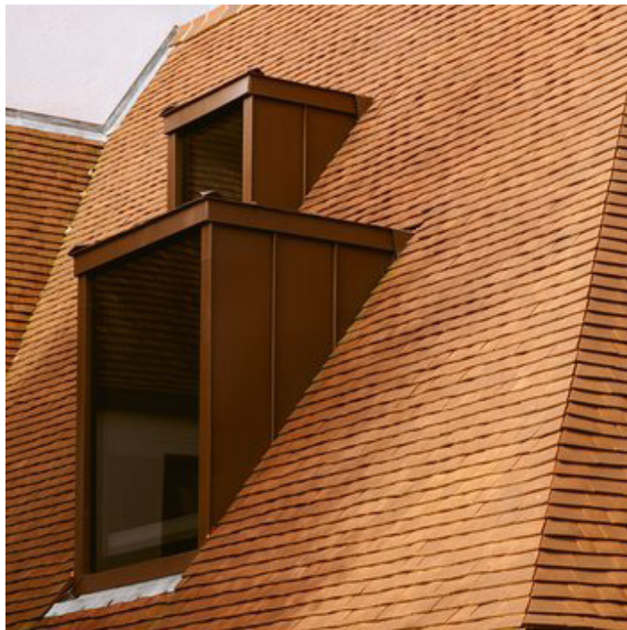
Example of Materiality Combination Zinc clad dormer window and clay roof tiles
