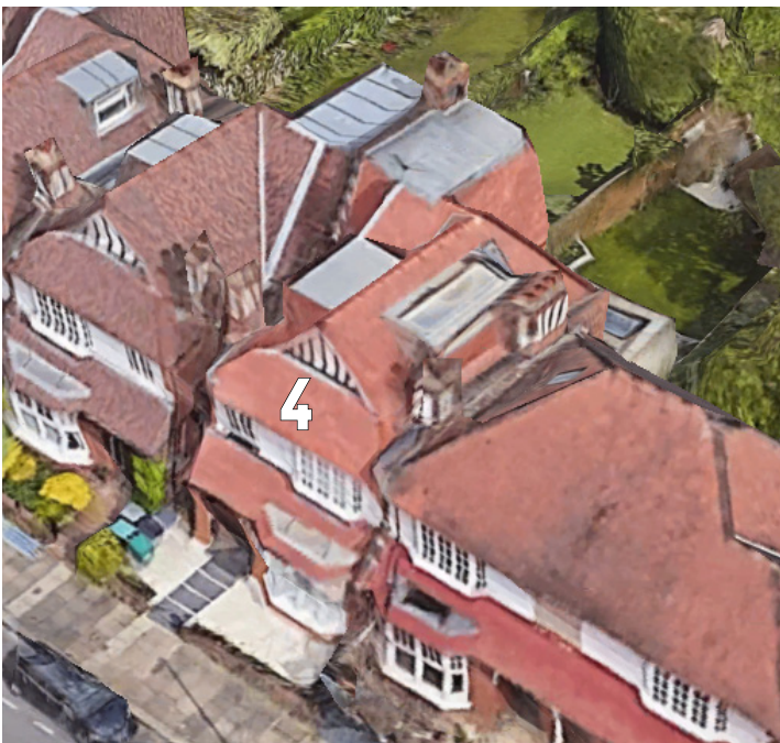
No. 4: Construction of two dormer windows a velux and a new air condition unit to be created at roof level.
