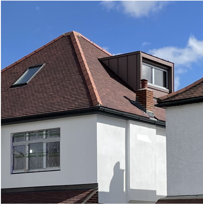
Zinc Dormer An example of a built dormer in red zinc with clay tile completed by Lineworks Architects and Portico Design & Build
