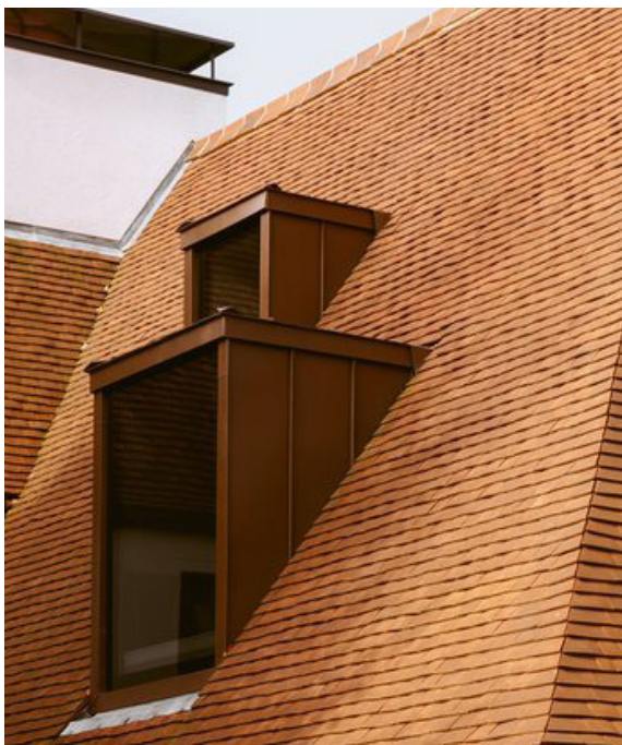
Example of Materiality Combination Zinc clad dormer window and clay roof tiles
