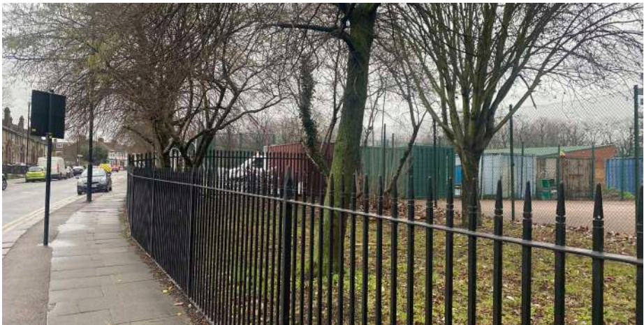
Railings for removal will be re-used
