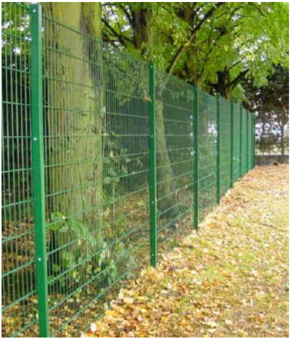
Visually permeable weld-mesh style fence along Park View Road set within existing tree line (2.1m high) colour to be black/grey
