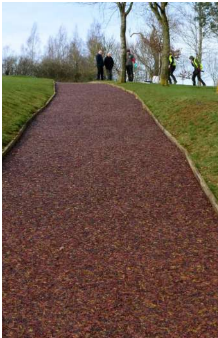
Northern play area safety surface - Rubber mulch safety surface
