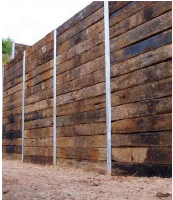
Reclaimed timber sleepers slotted into steel beams to form boundary up to 2.4m high softened by new trees and climbing plants
