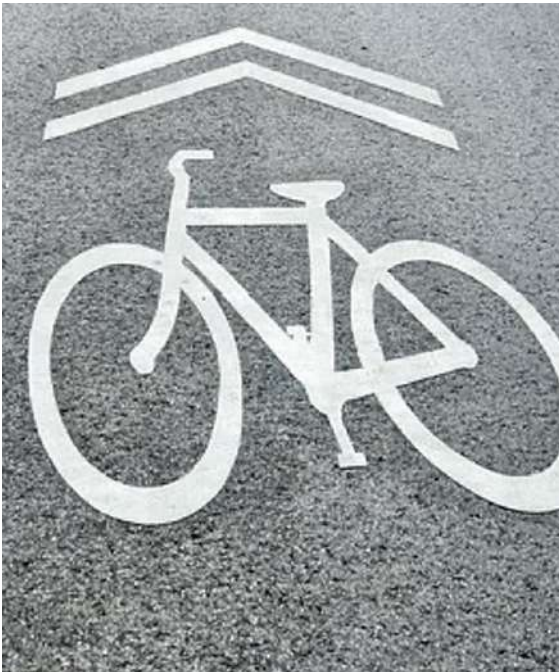
Thermoplastic signage to hard-surfacing routes (cycle paths, distance markers etc)
