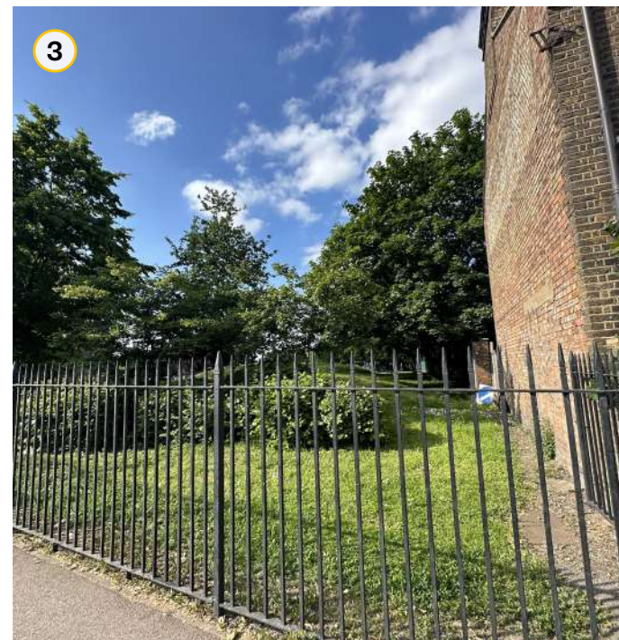
Photo 3 of existing railings, approximately 1.2m high to be removed to create new southern park entrance
