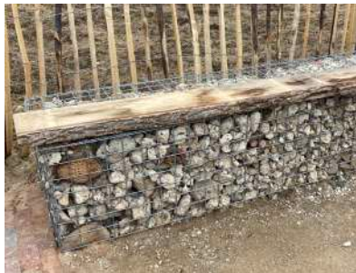
Hardcore for gabion baskets
