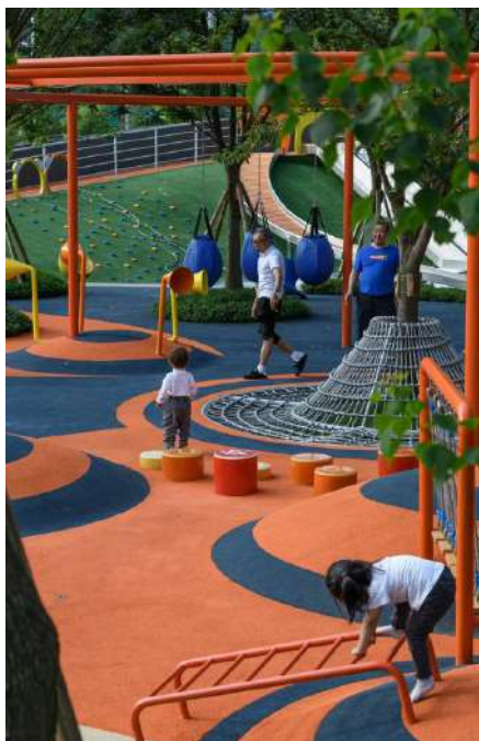
Southern play area safety surface - Wetpour safety surface
