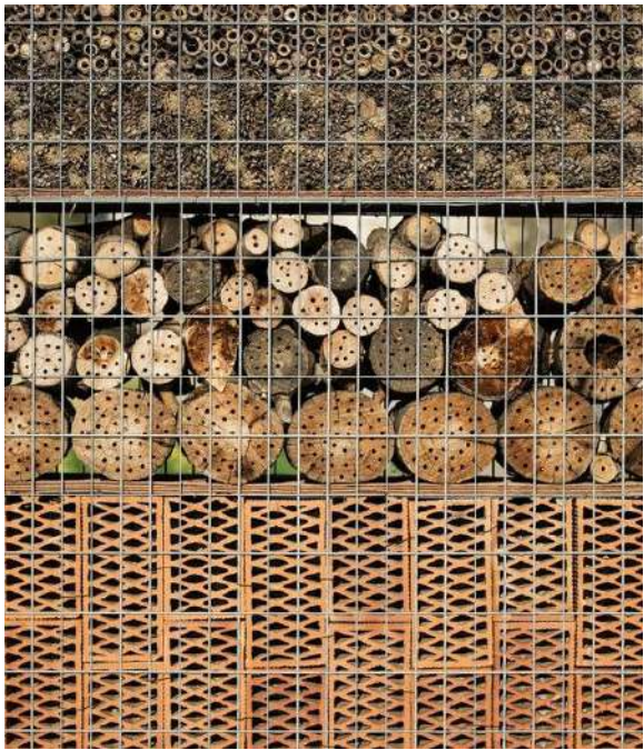
Galvanised steel gabion basket backfilled with site-won materials such as concrete, brick, setts and other wildlife-friendly components such as tree timbers (2.1m high)
