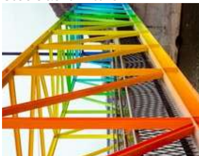
Steels re-primed and painted
