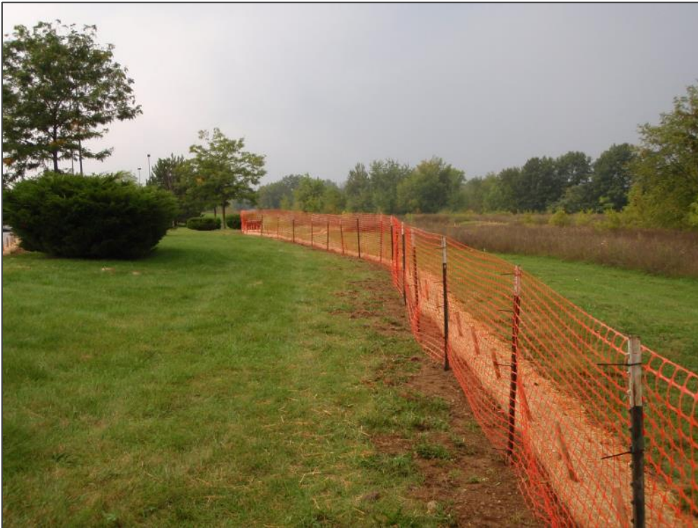
Example of lower specification barrier
