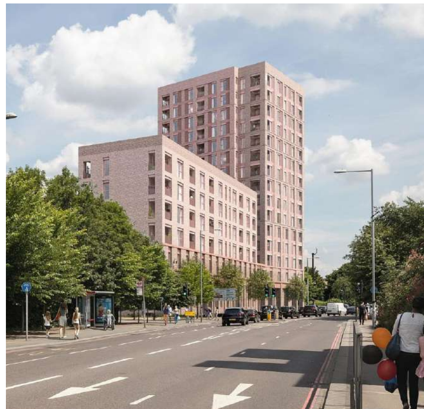
Welbourne District Health Centre and Walter Tull House
