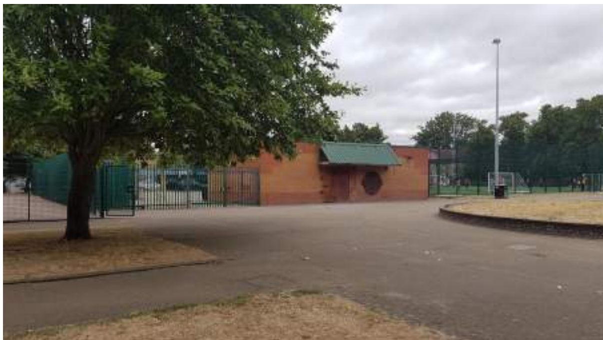
Figure 4.2 Eastern facade of Building two
