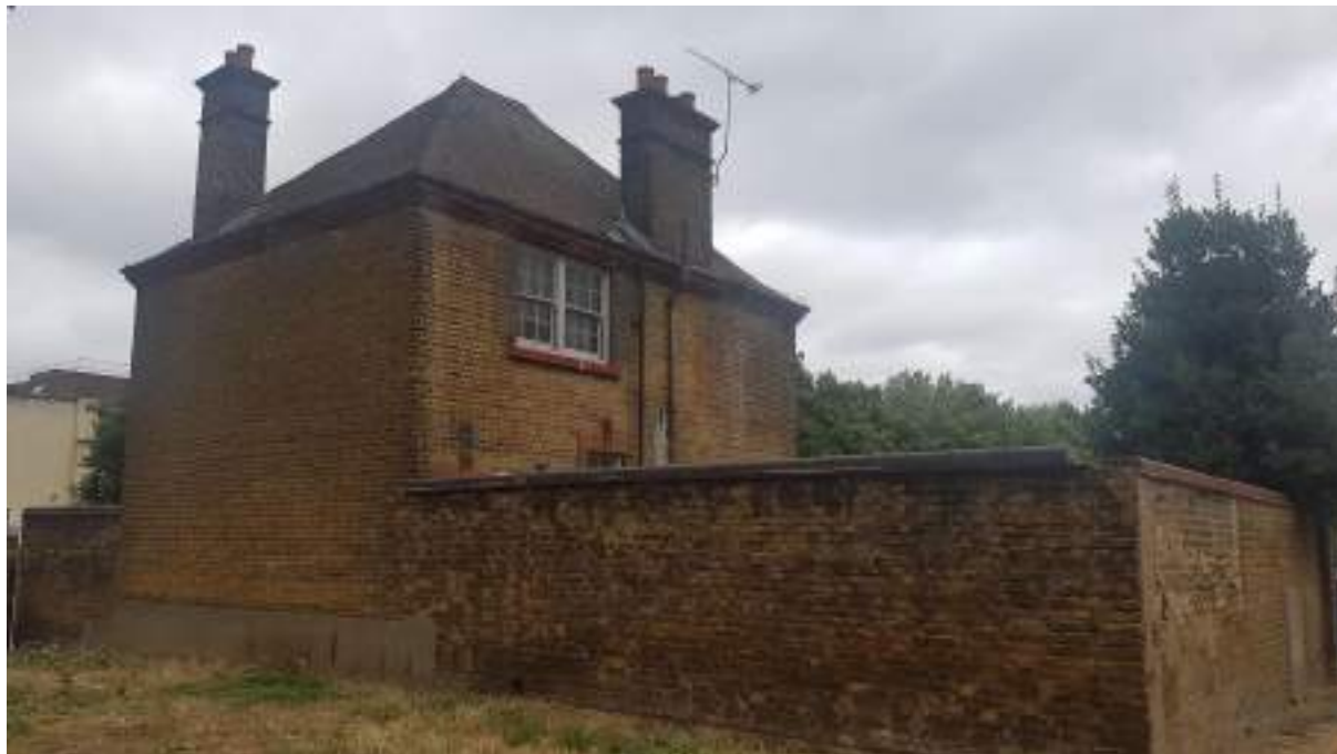
Figure 4.3 South and eastern facade of Building three
