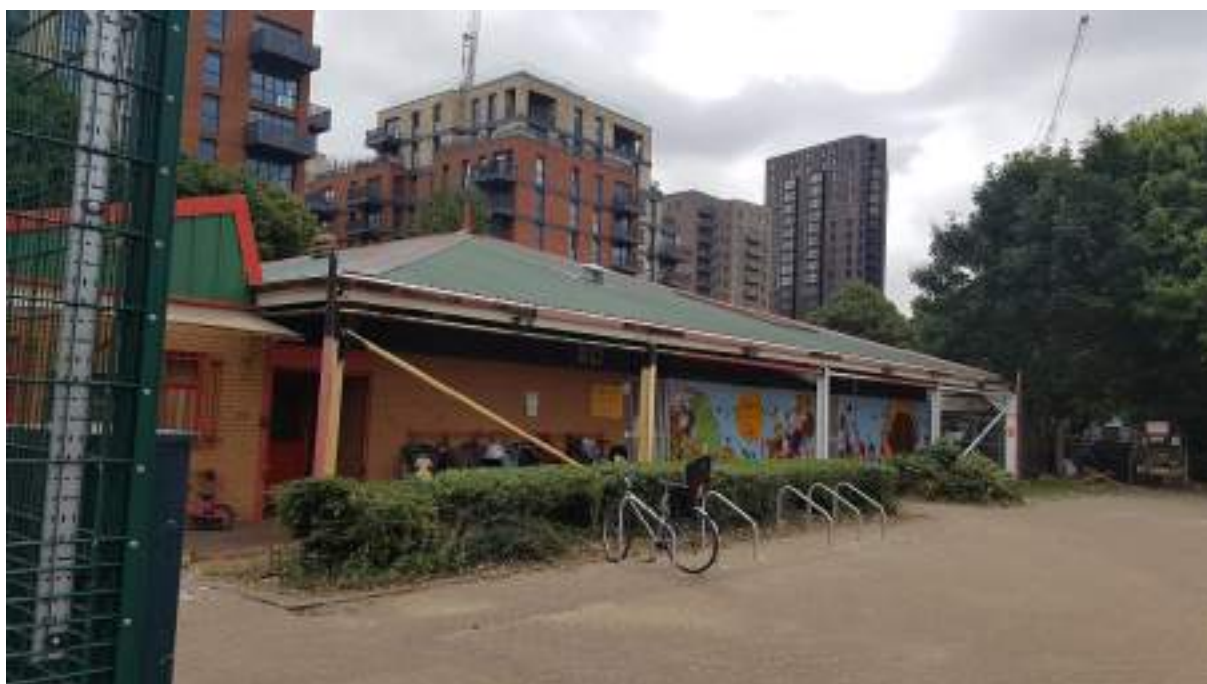
Figure 4.1 Western facade of Building one
