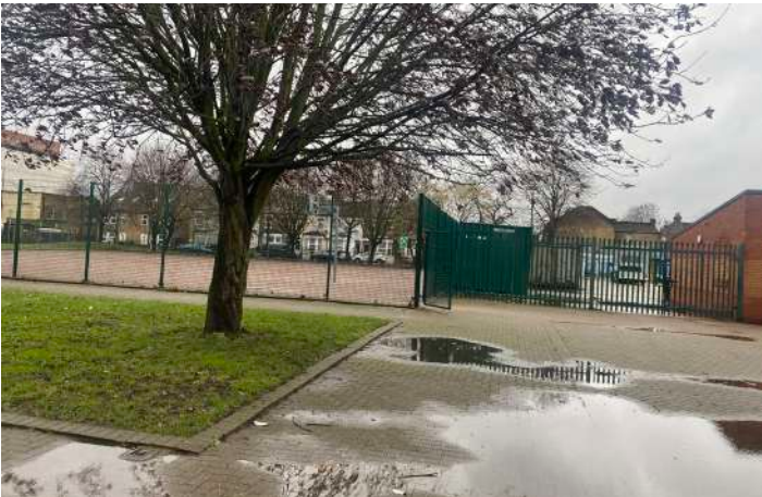
Large areas of existing impermeable surfaces require drainage infrastructure to be regularly maintained
