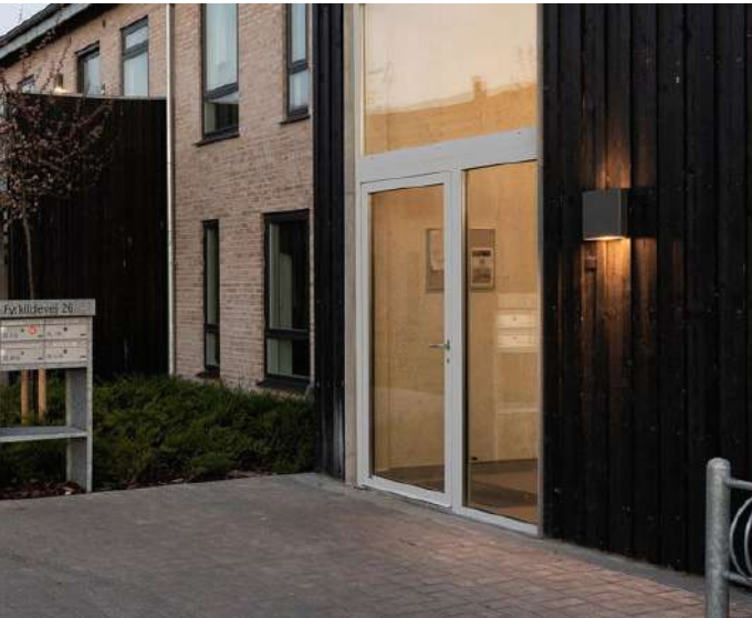
Low glare and residential aesthetic lighting support identity and character
