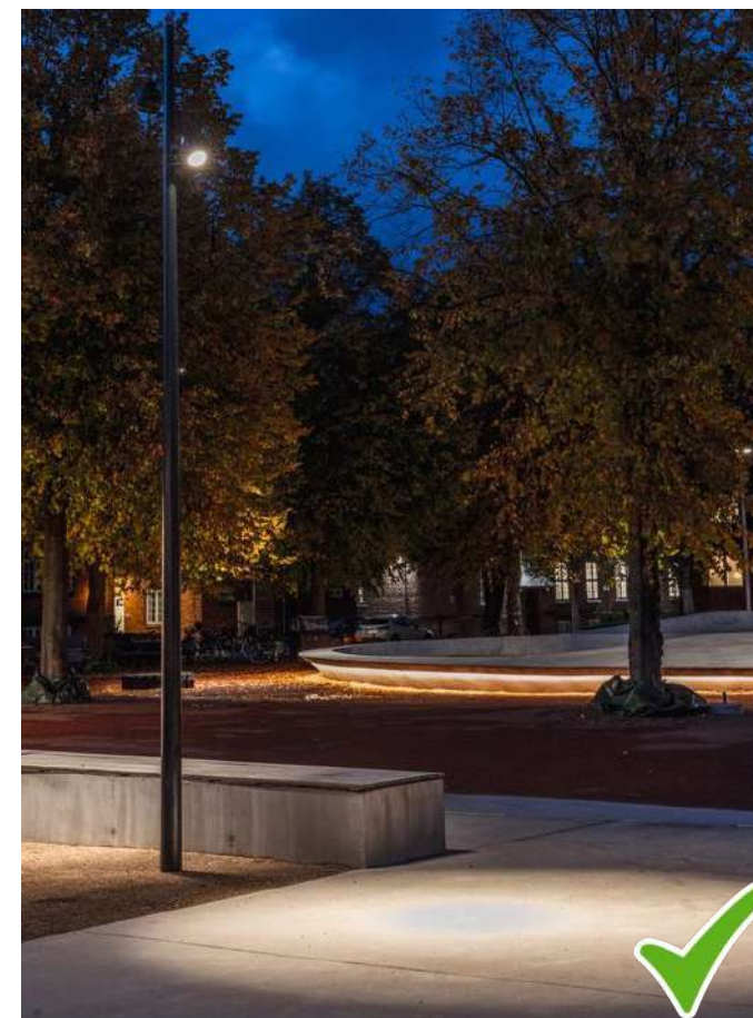
Controlled aiming and light distribution avoids unwanted light spill
