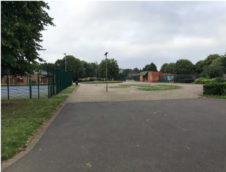
View of southern portion of site with tennis courts in foreground and existing council depot to the right – Looking south
