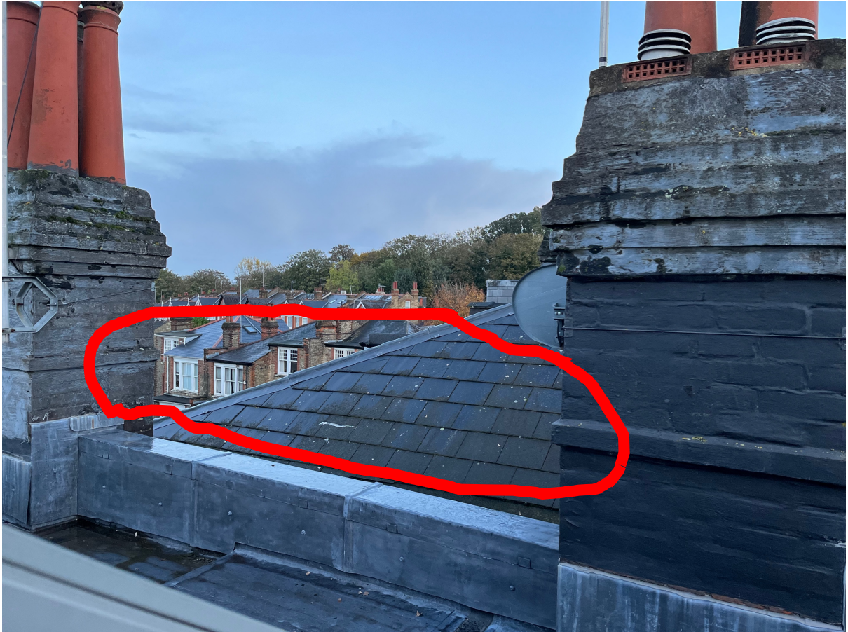
Figure 1: Proposed location of the balustrade. Photo taken from the Velux window in the living room of 21D Methuen Park. 4 November 2023.
