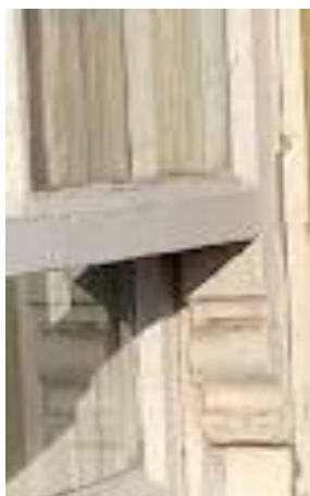
Top sash detail Decorative horns 112mm
