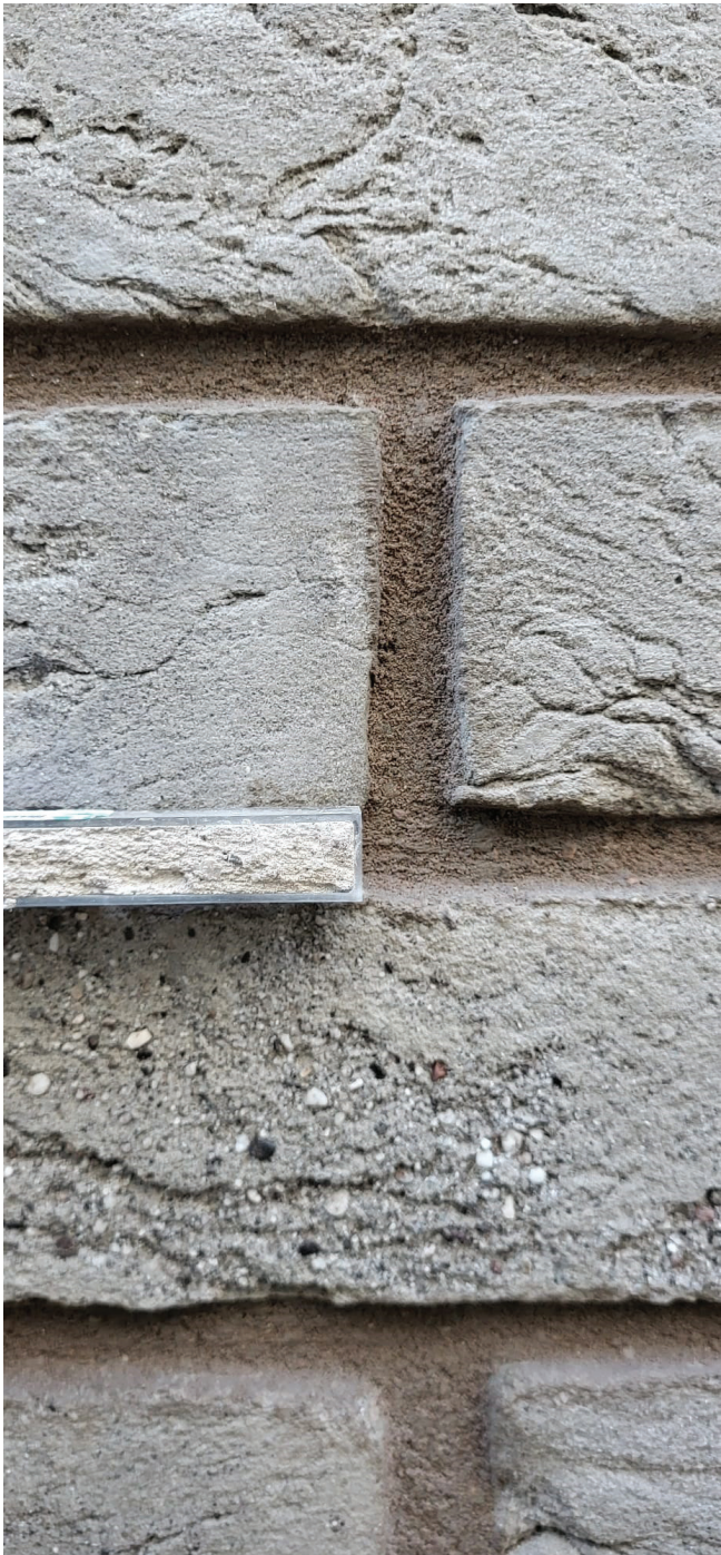
03 Proposed brick + lime mortar samples Note: the mortar between the bricks has not cured completely hence why it shows a draker colour. The mortar sample confirms the final colour.
