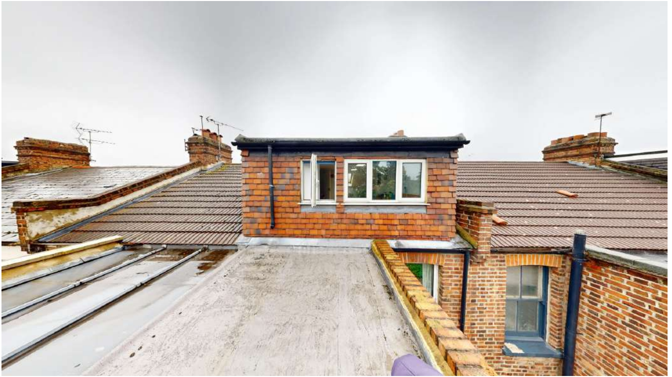
View - Existing Roof Extension
