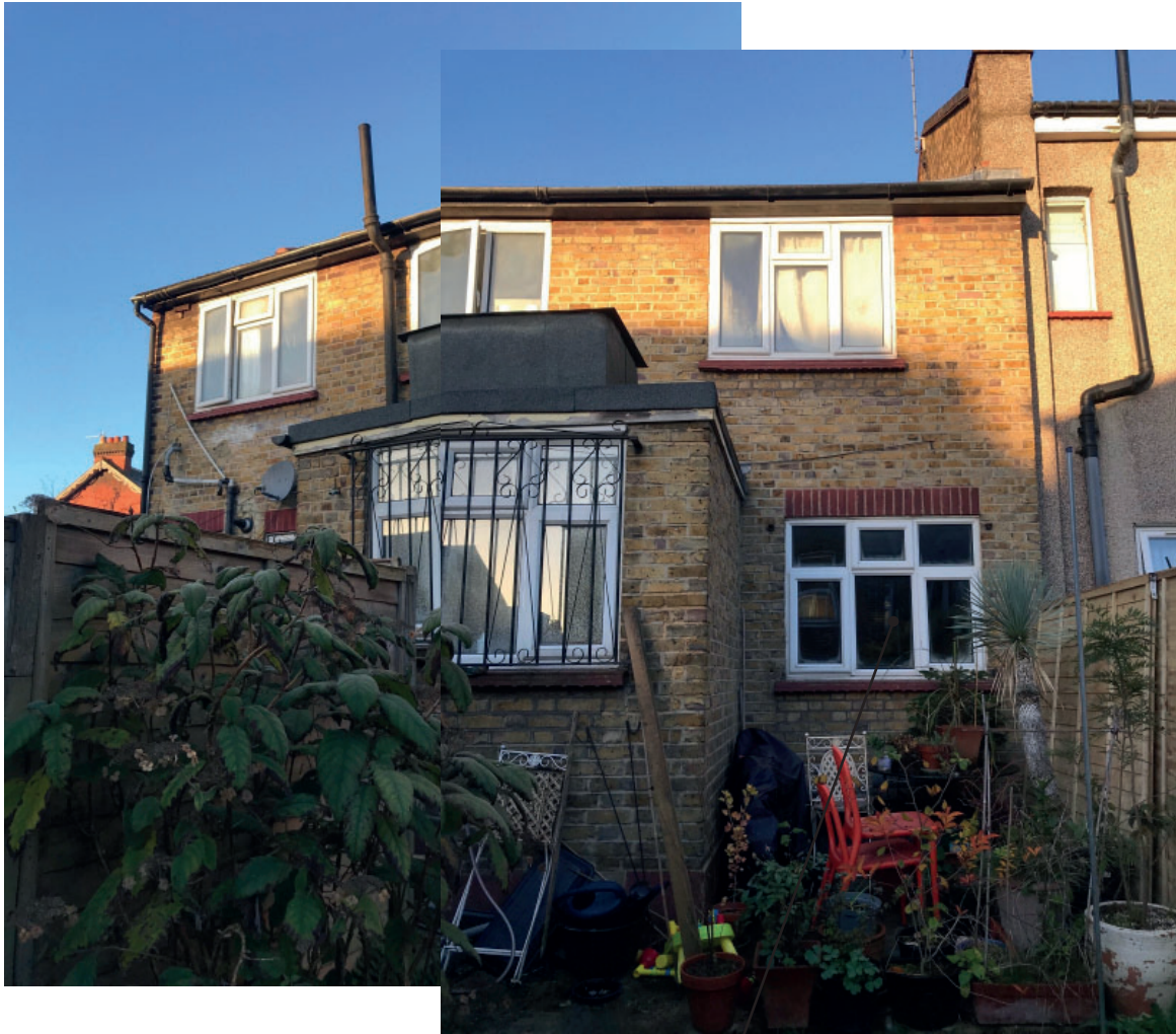
Picture 03: Rear elevation
