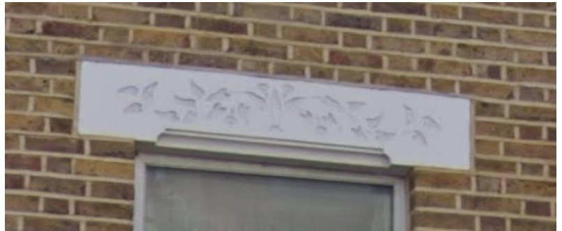
Detail of Lintels to be replicated
