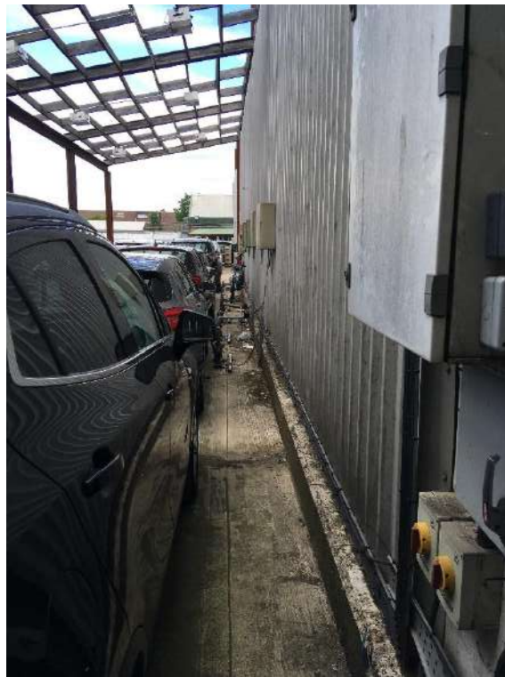
Photograph 1 – cars parked over 5 underground storage tanks, (disconnected)
