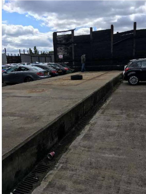
Photograph 3 – Raised concrete plinth in the centre of the Site. Assumed to formerly house compactor.
