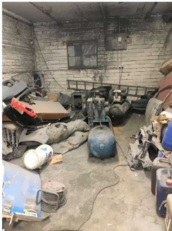
Photograph 6 – Northern Building used for storage, compressed gas pump visible.
