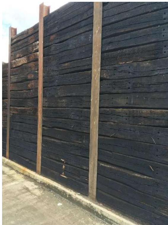
Photograph 2 – Reclaimed railway sleepers, used as retaining walls around Site
