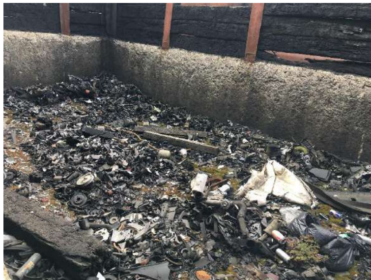
Photograph 4 – Central inaccessible compound, with evidence of Sites former use with waste car parts present.
