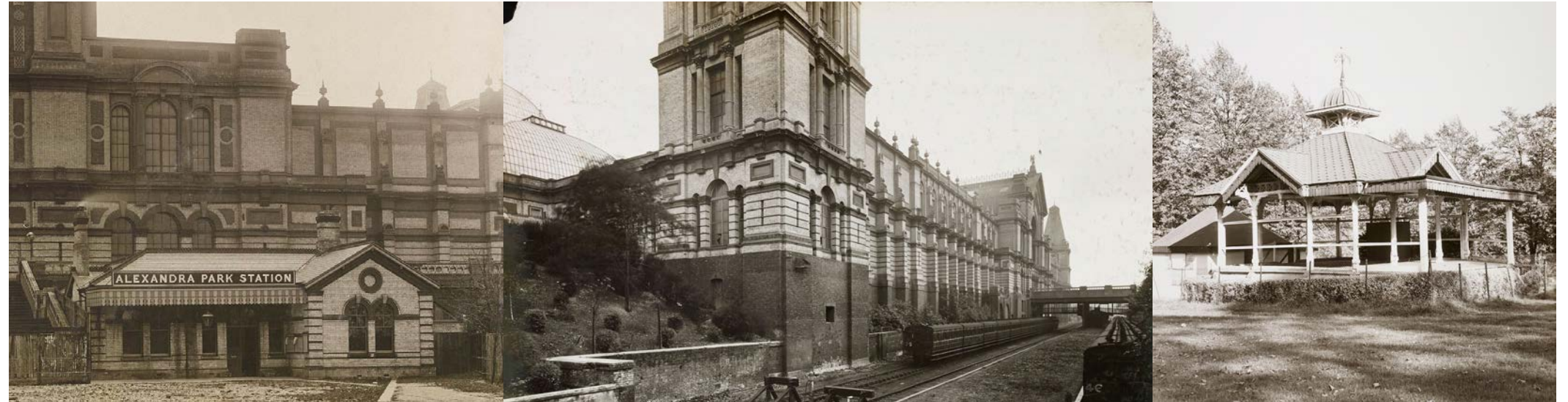
Architecture of Alexandra Palace
