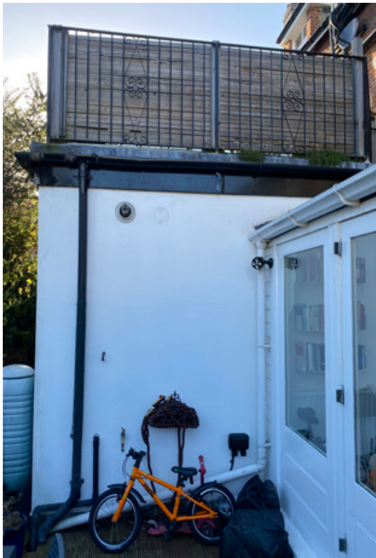
03 Rear facade - screened terrace above No.7b's masonry extension
