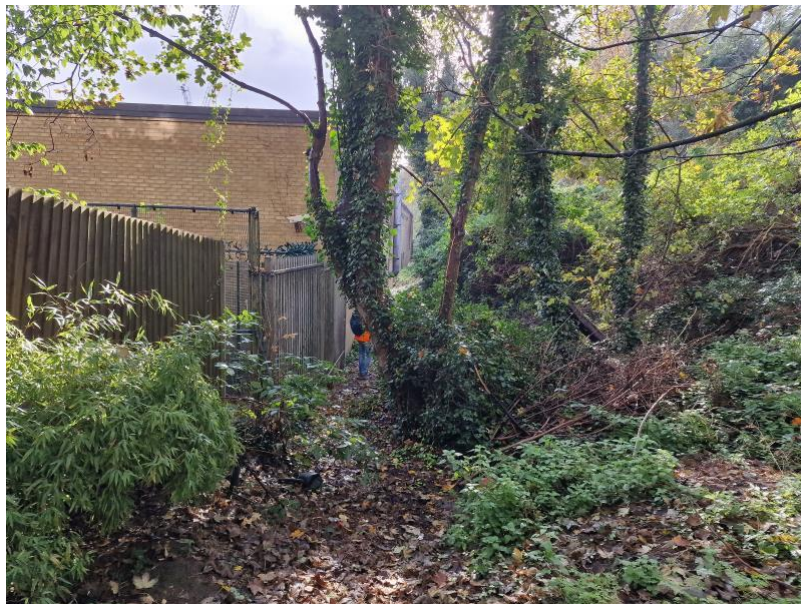
Figure 1: T12 in relation to the north-western corner of the police base building.
