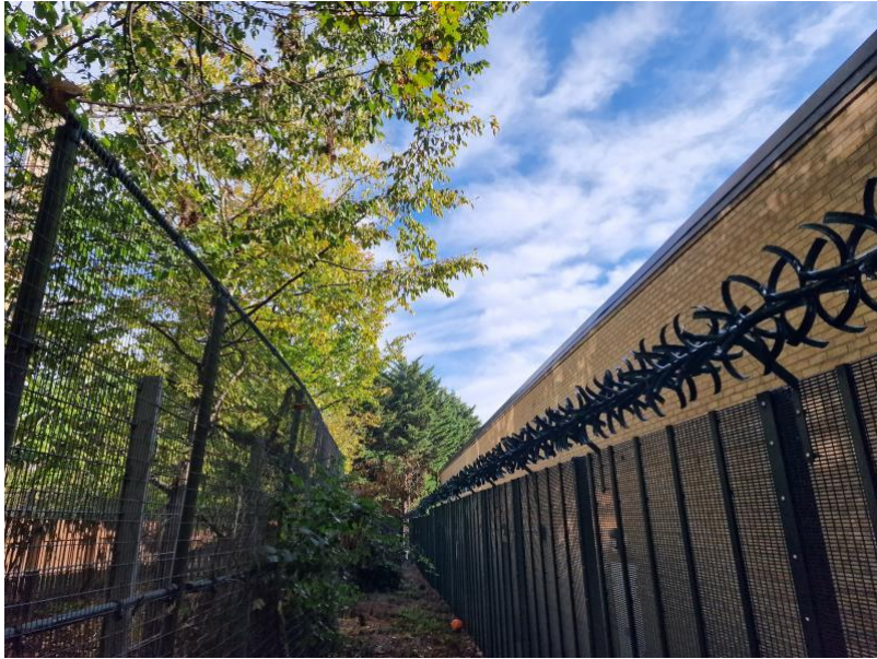
Figure 2: Crown clearance between the police base building.
