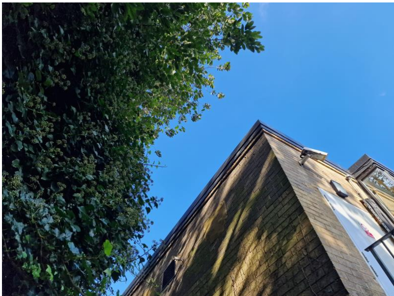
Figure 7: Upper crown clearance between the police base building and T21.
