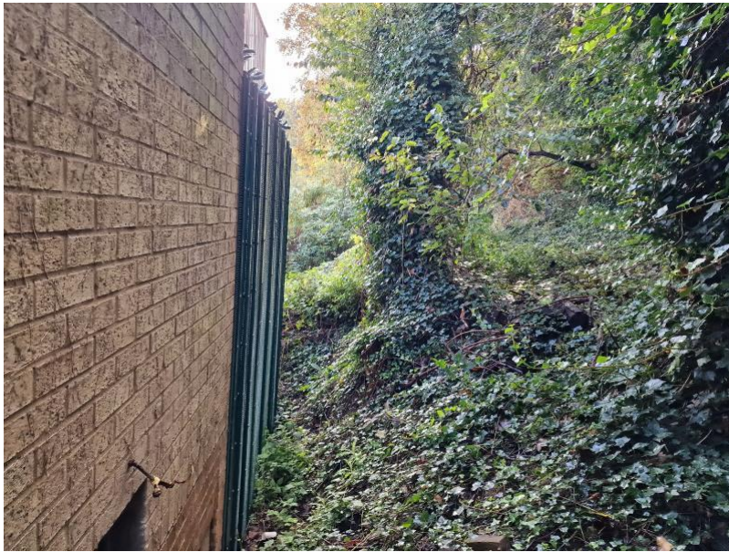
Figure 8: T22 located south of the south-western corner of the police base building.
