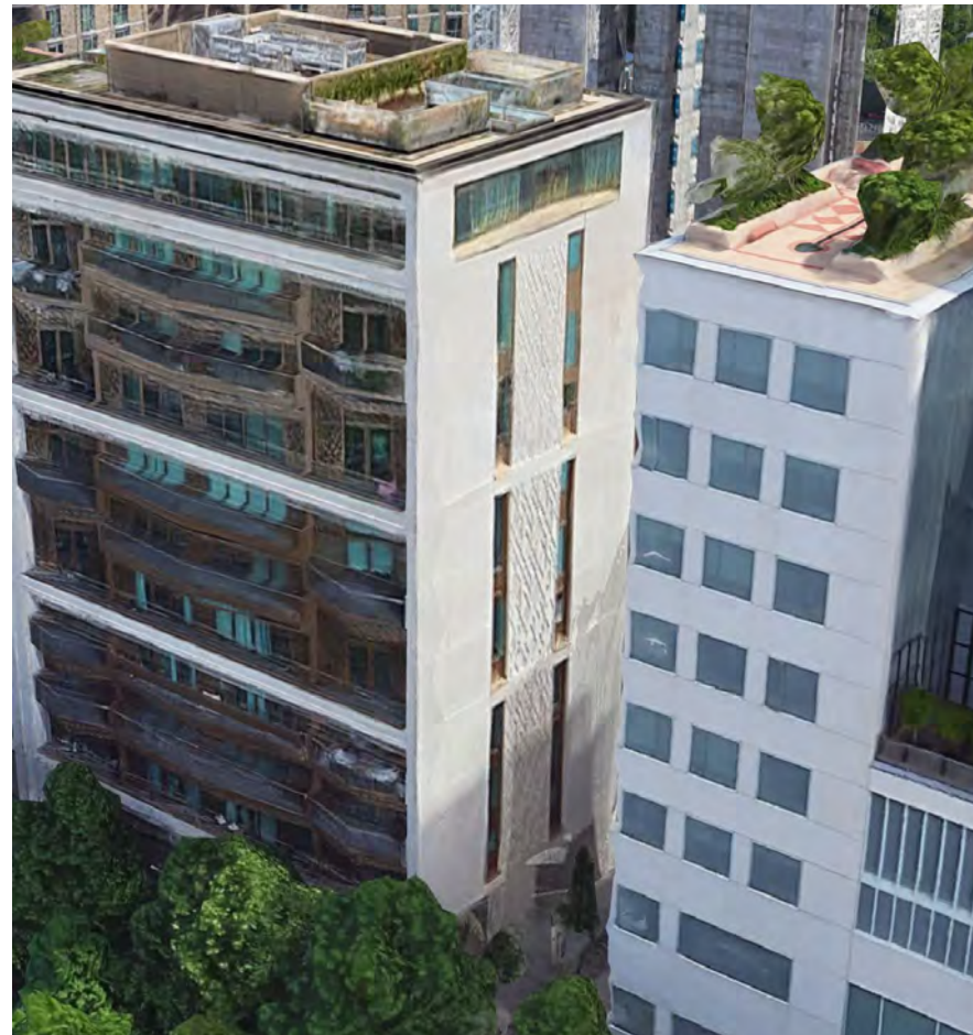
FIGURE 11 - EXAMPLE OF EXPOSED FLANK WALLS FORMING A GAP WITH LIMITED WINDOWS
