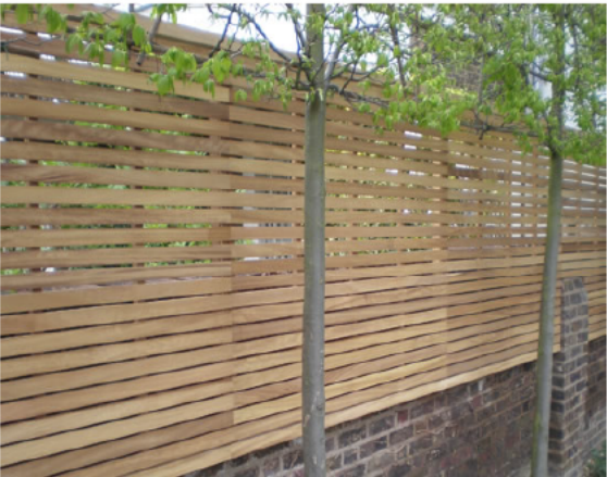
An example of timber horizontal screens and brick wall
