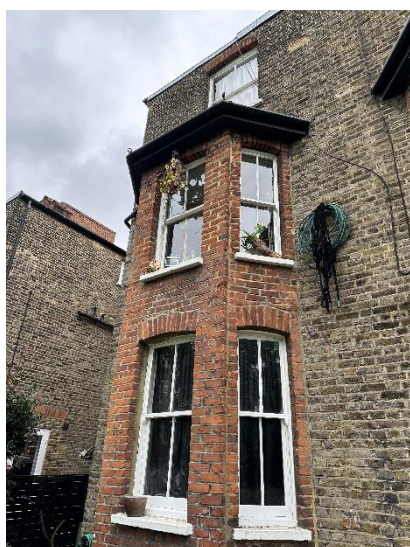
Figure 6: 78 Cecile Park Rear Elevation Windows
