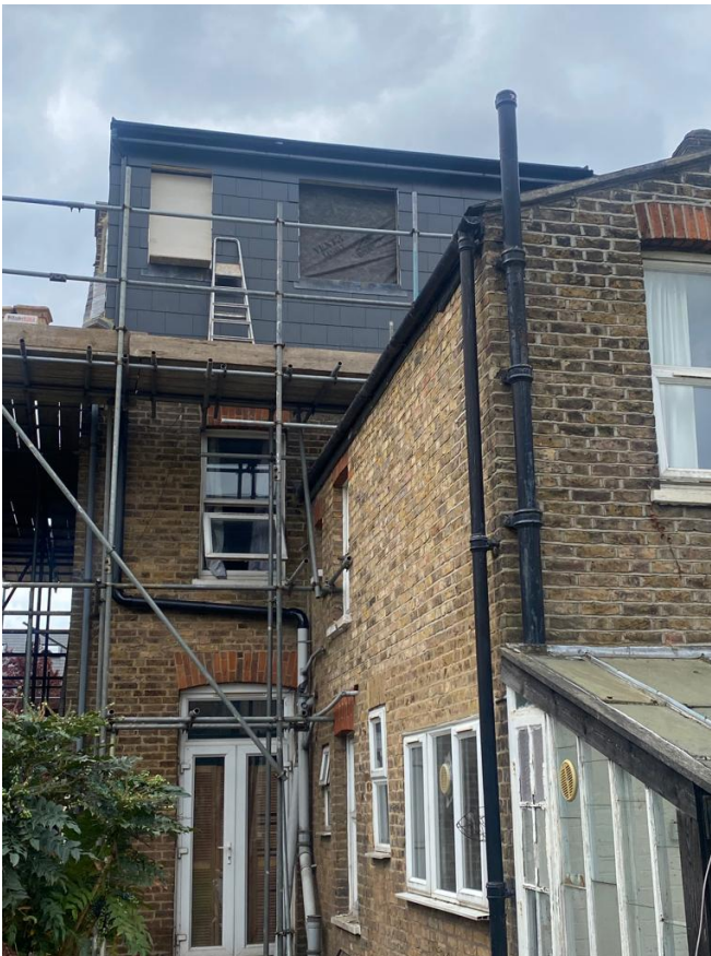
Rear view with loft dormer constructed
