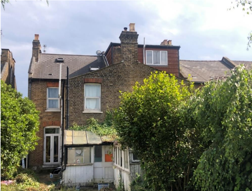
Rear view prior to construction of loft.
