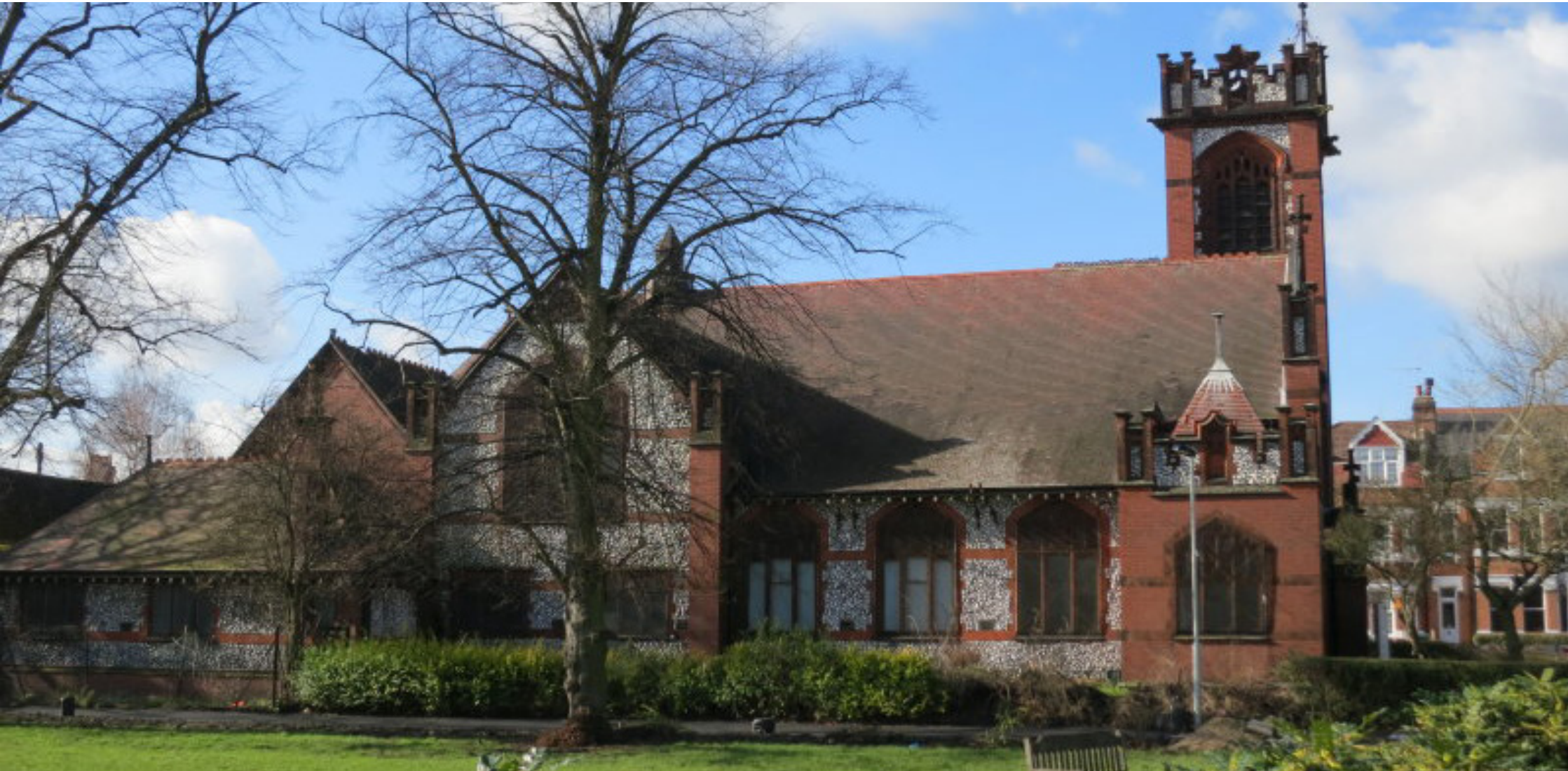
Existing building on Site
