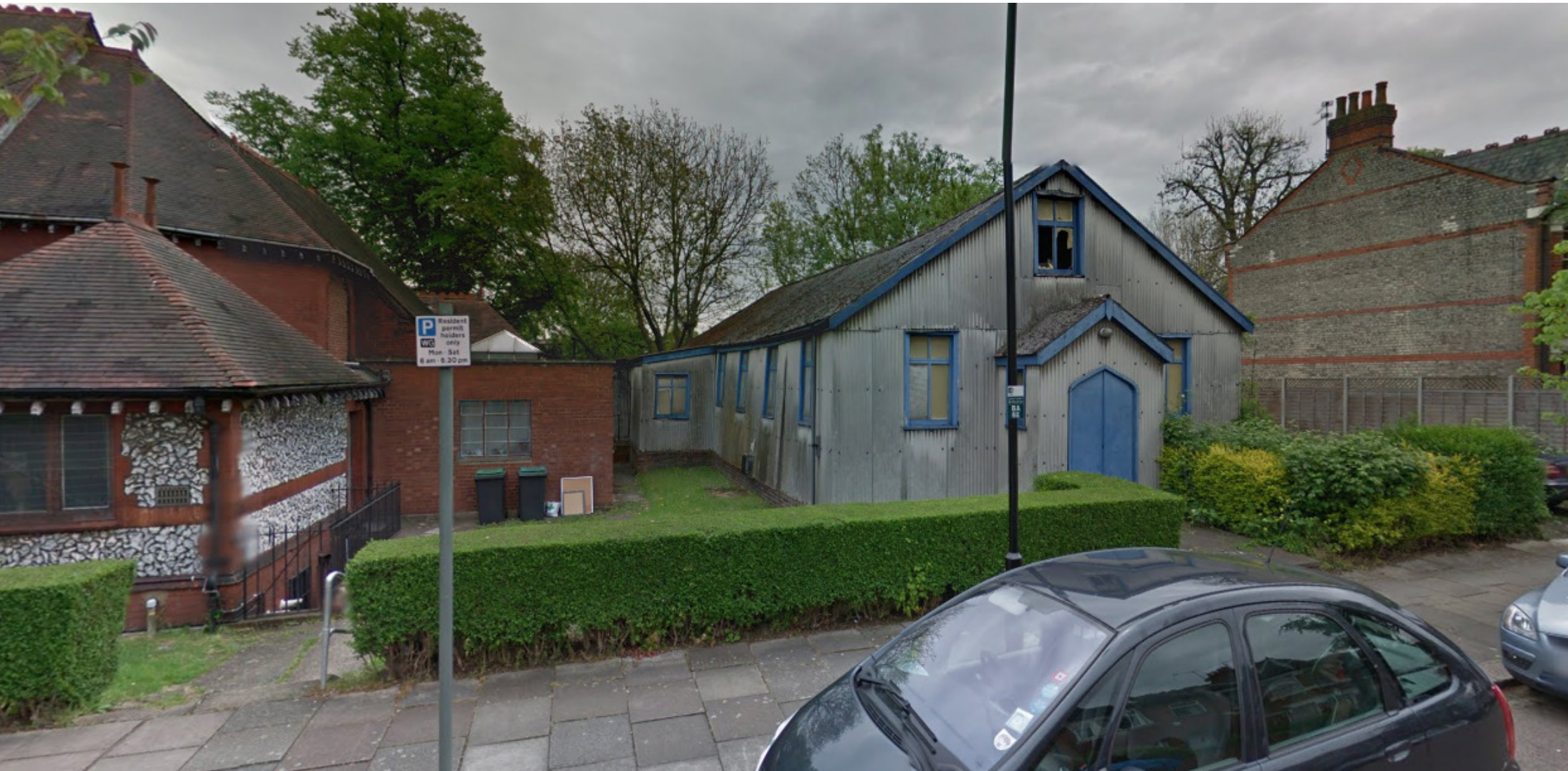
Existing tin tabernacle on Site
