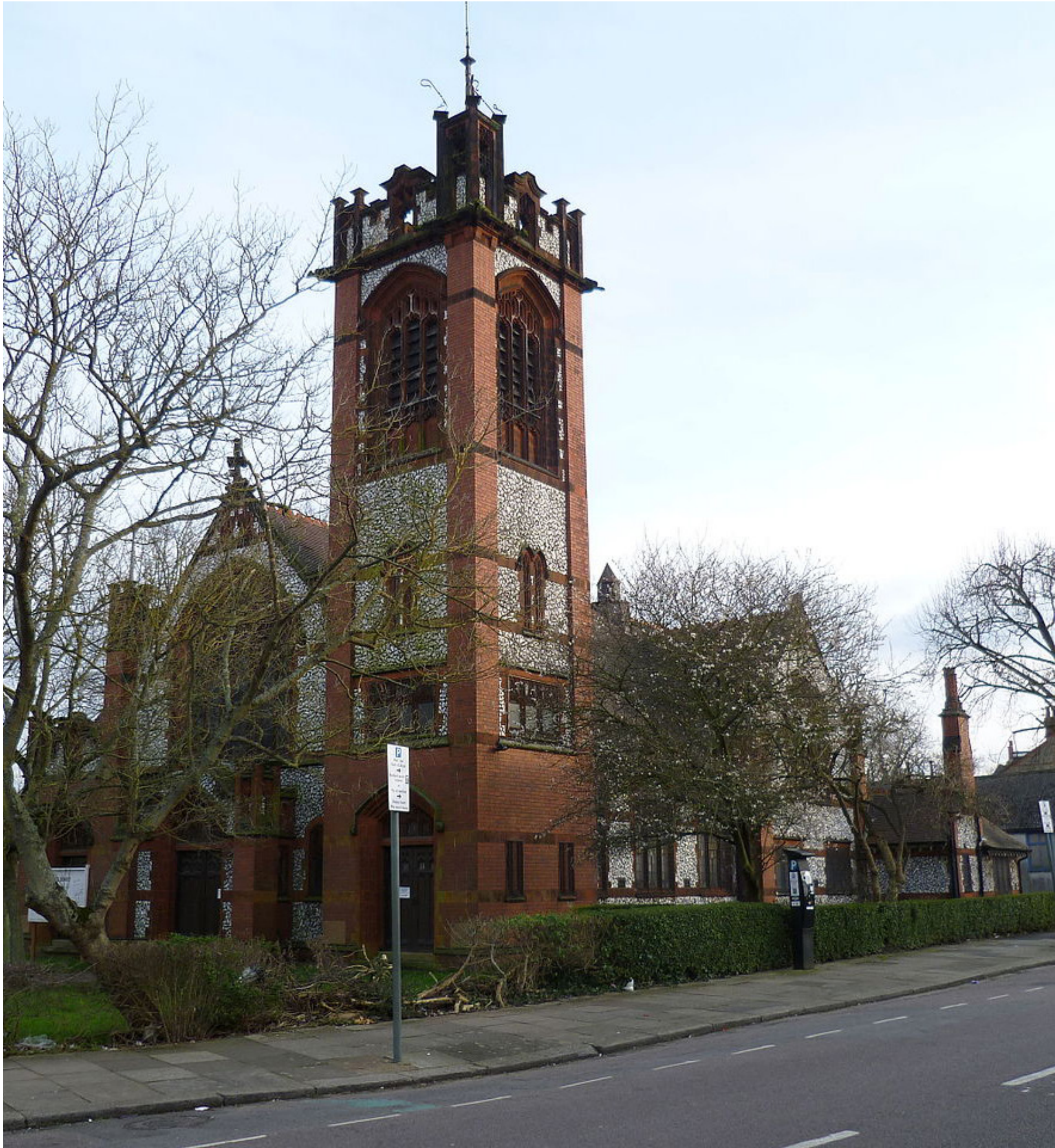
Existing building on Site
