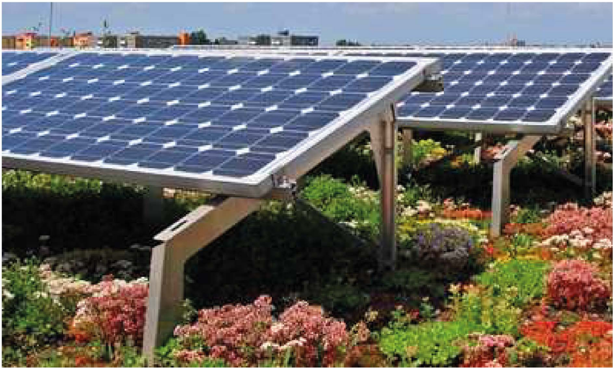
Church Green Roof & Residential green roof with PV Panels
