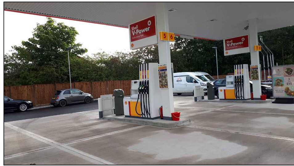
Situ concrete forecourt surfacing with light brush finish and dispenser island arrangement
