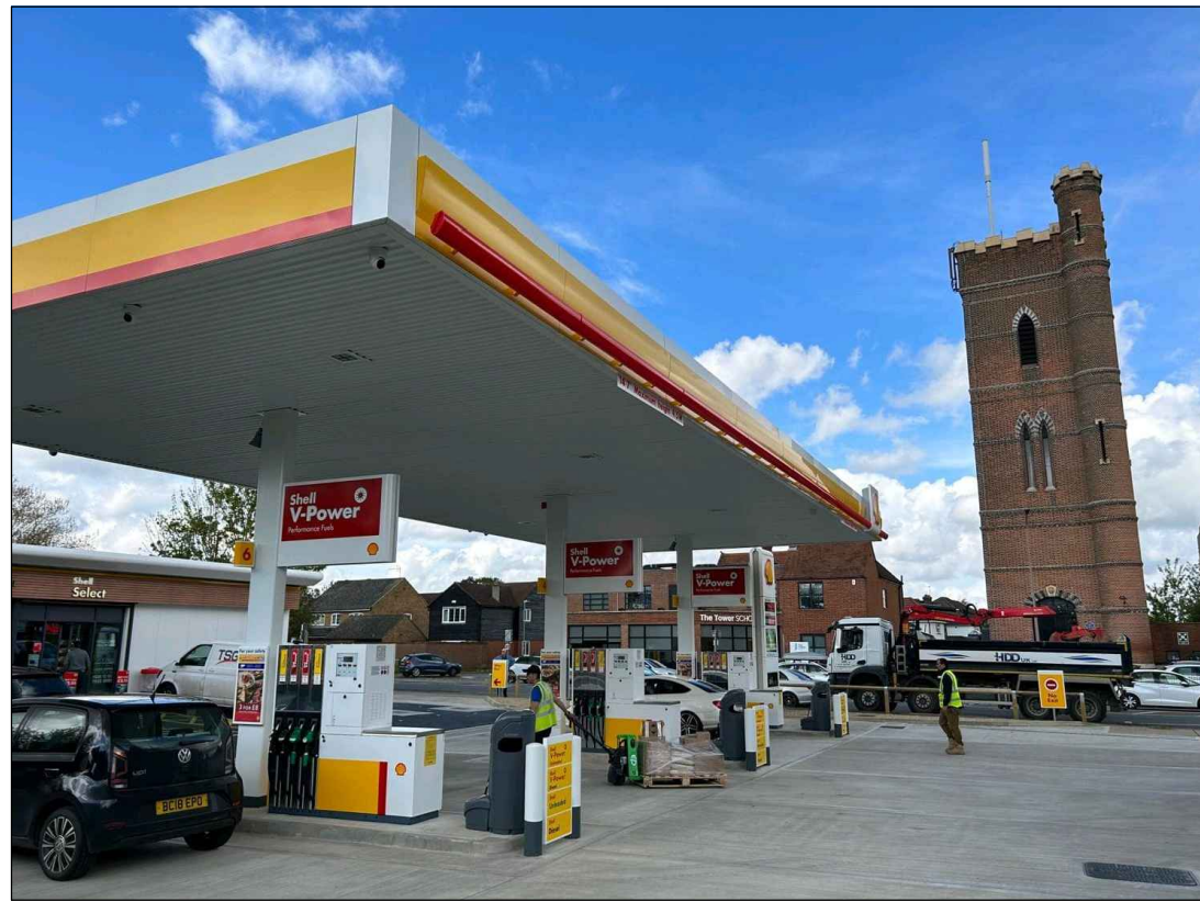
Steel framed forecourt canopy in painted steel stricture and fascias with white profiled steel roof sheet and soffit underlining finish
