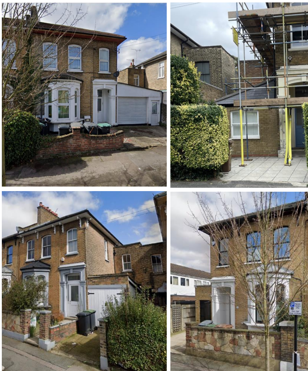
Figure 1: Google Street View (2018) images of garage extensions at no. 16 Bedford Road (top left), no. 29 Bedford Road (bottom left) and no. 31 Bedford Road (bottom right). Photograph of the side extension at no. 23 Bedford Road (top right).
