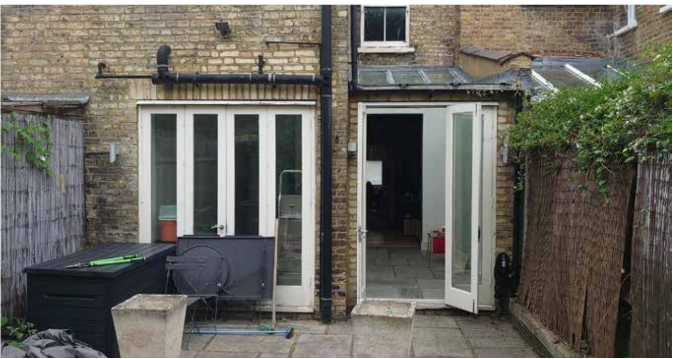
Existing Infill Extension (rear)
