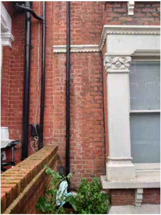
Existing front facade brickwork
