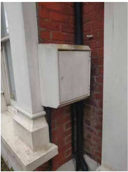
Existing front garden services
