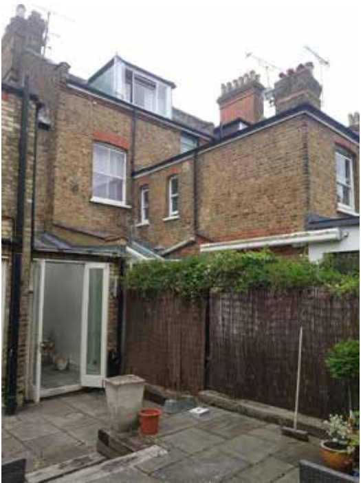
Existing Infill Extension (rear)
