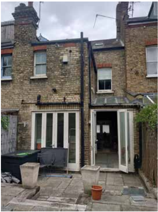
Existing rear facade
