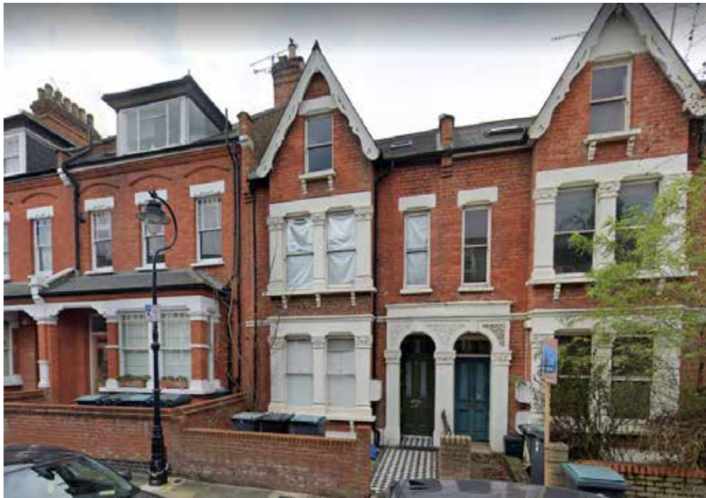
Front View of 11 Drylands Road
