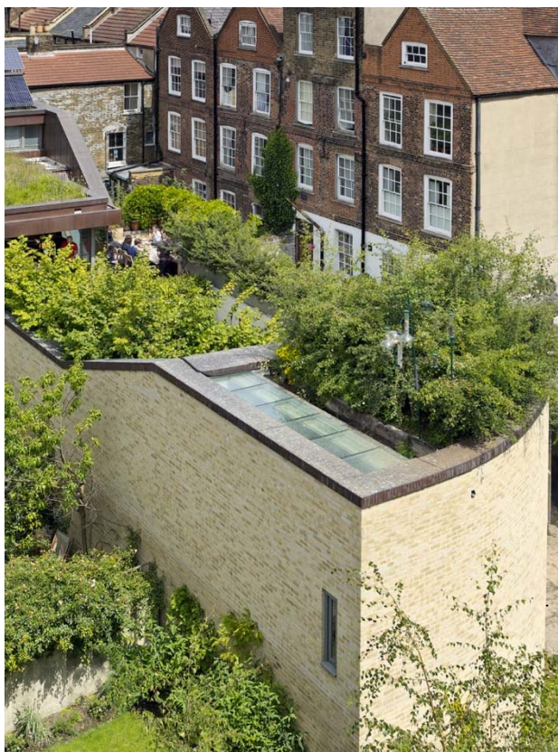
Roof for single storey part of building
