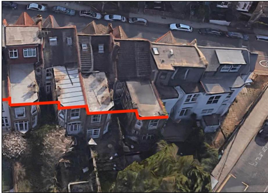
Figure 6: The rear elevations step down towards Albert Road.
