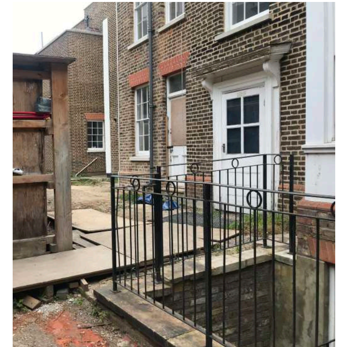
FIGURE 7. Land to the Rear of No. 794 looking South
