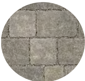
ST_04 Parking bays: permeable concrete paving
