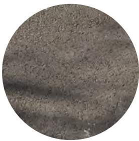
ST_01 Carriageways: asphalt
