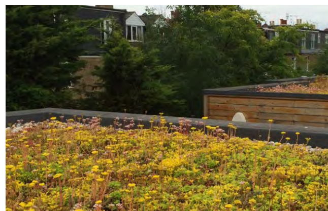
Extensive sedum roof
