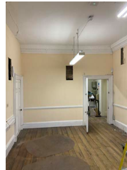
Existing decorative plasterwork in first floor room F8
