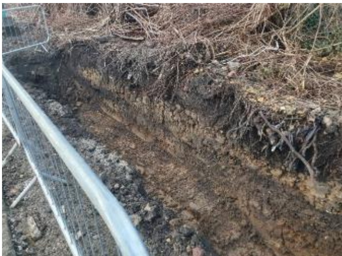
Image 33: Root Barrier Works
