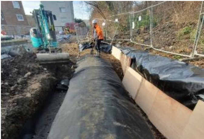
Image 39: Root Barrier Works
