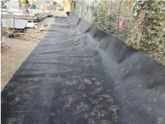
Image 43: Root Barrier Works
