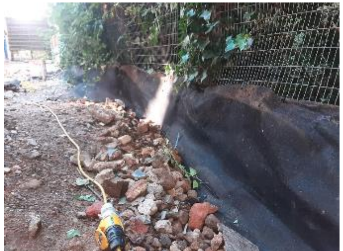
Image 466: Root Barrier Works
