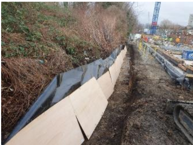
Image 33: Root Barrier Works
