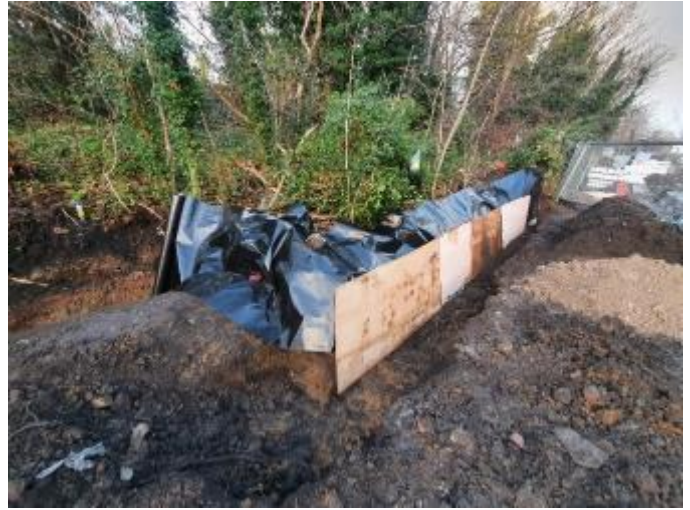
Image 38: Root Barrier Works
