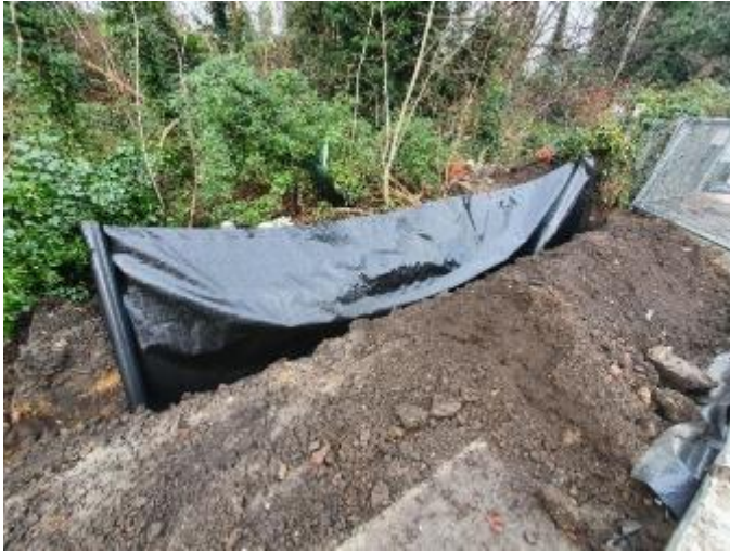
Image 37: Root Barrier Works
