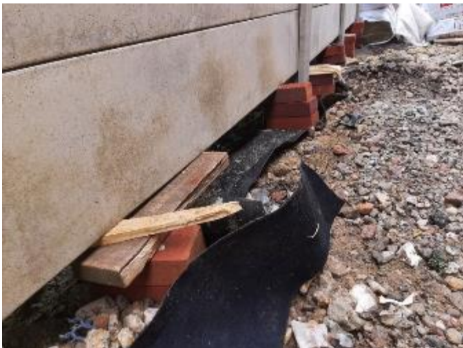
Image 45: Root Barrier Works
