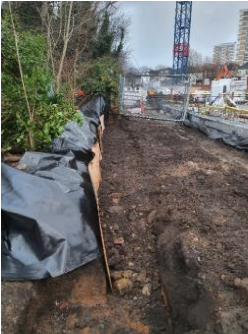
Image 39: Root Barrier Works
