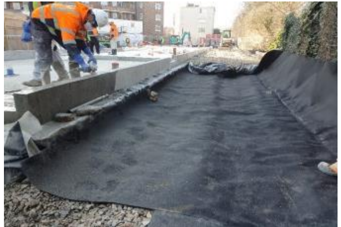
Image 40: Root Barrier Works
