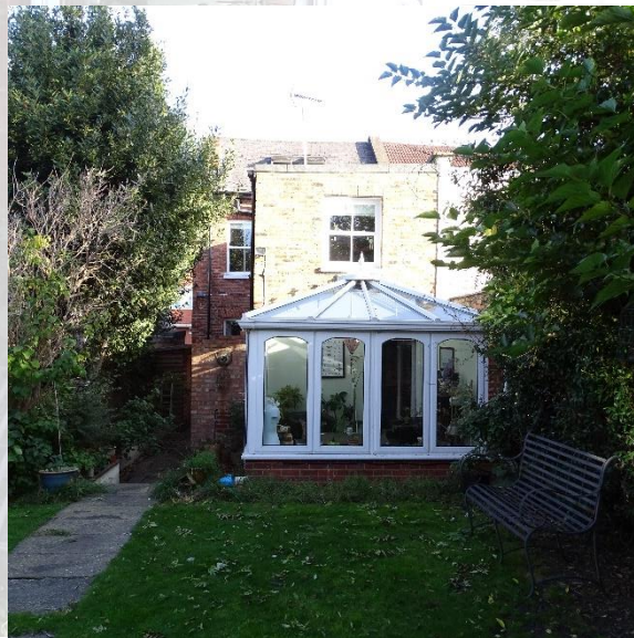
View of the rear of 15 Caxton Road
